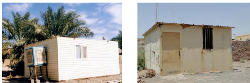
Figure 5: Prefabricated units assembled in the yard of destroyed houses (Source: Authors).
