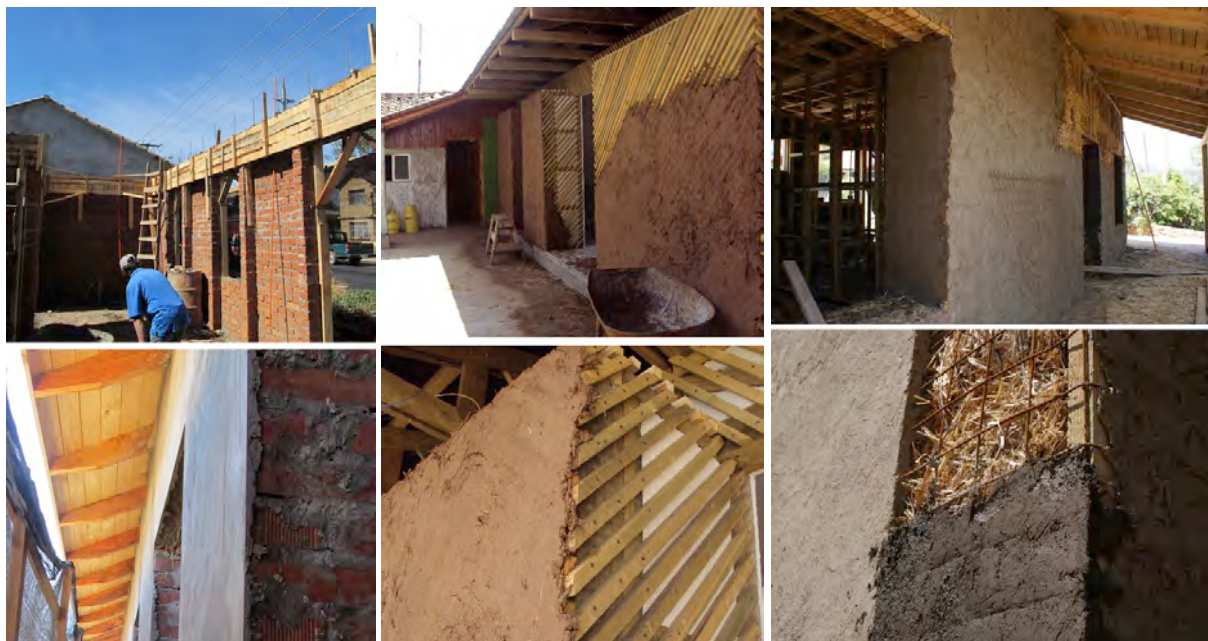
Figure 8: Building techniques used in housing reconstruction for heritage areas. From left to right: a) reinforced brick masonry; b) timber structure with clay plaster; and c) timber structure with straw bales in the façade and wood panels with clay in the rest of the walls. (Source: Author).
