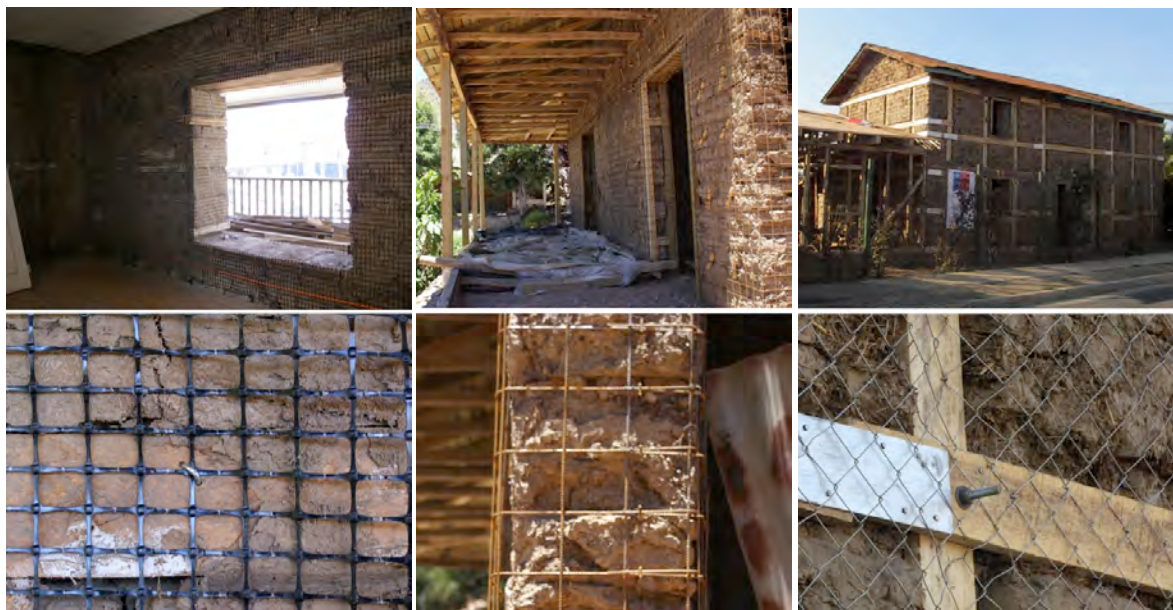
Figure 5: Reinforcements techniques. From left to right: a) geomesh used in Almahue (Source: author); b) metallic mesh in Lolol (Source: author); and c) timber reinforcements in Olivar (Source: F. Pérez, MINVU).
