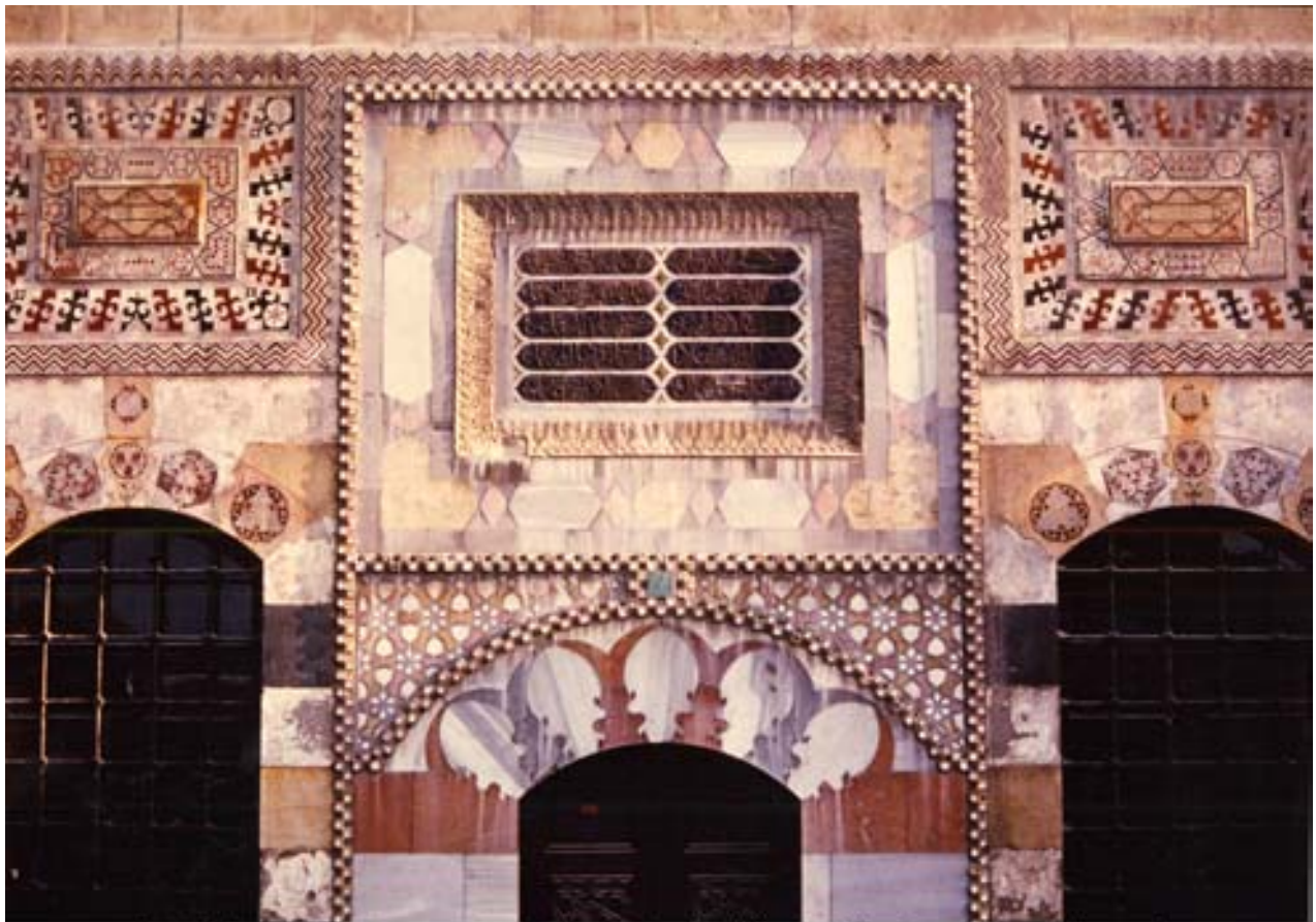
Details of the stonework and plaster infilling of the façade of the qa'a
