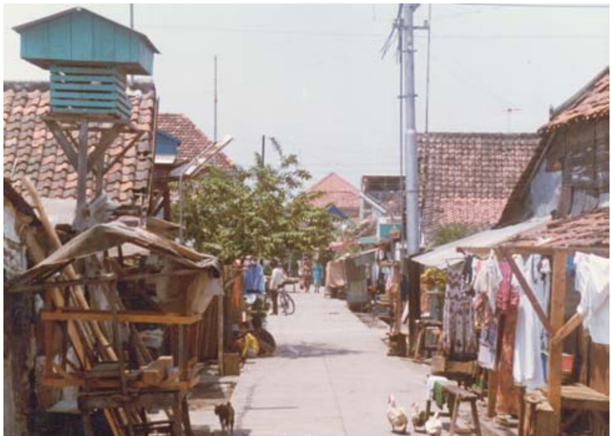
Foothpath and drainage system: after
