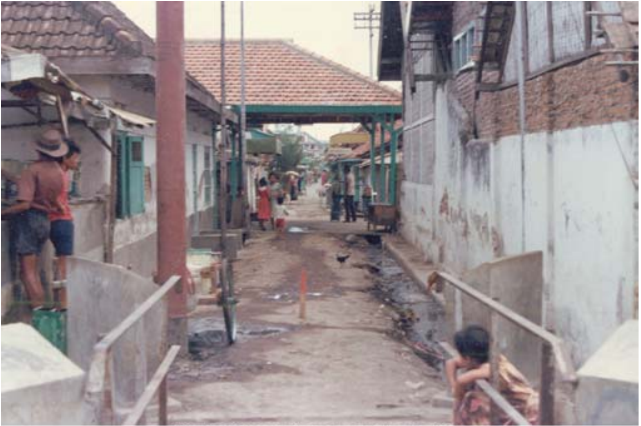
Foothpath and drainage system: before
