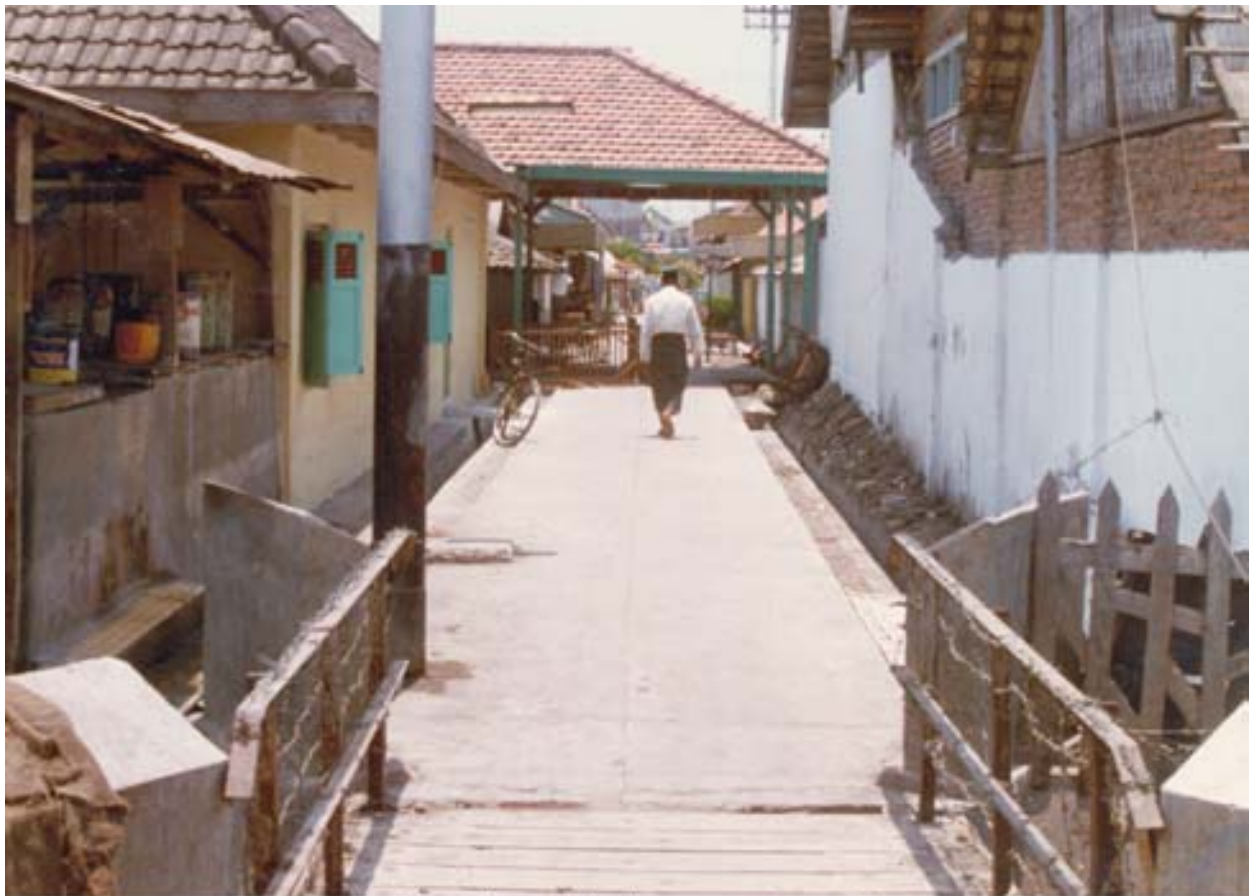
Foothpath and drainage system: after
