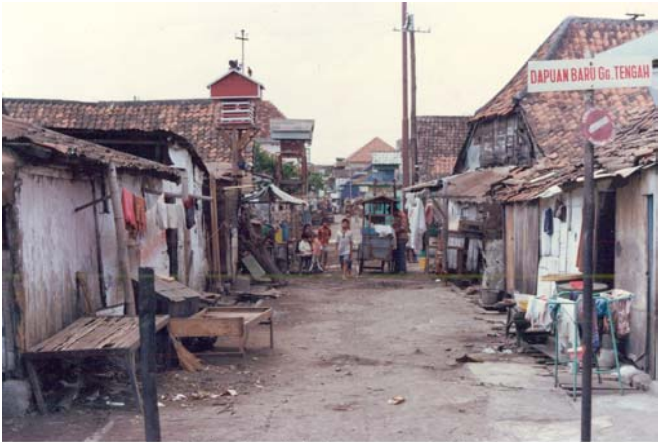
Foothpath and drainage system: before
