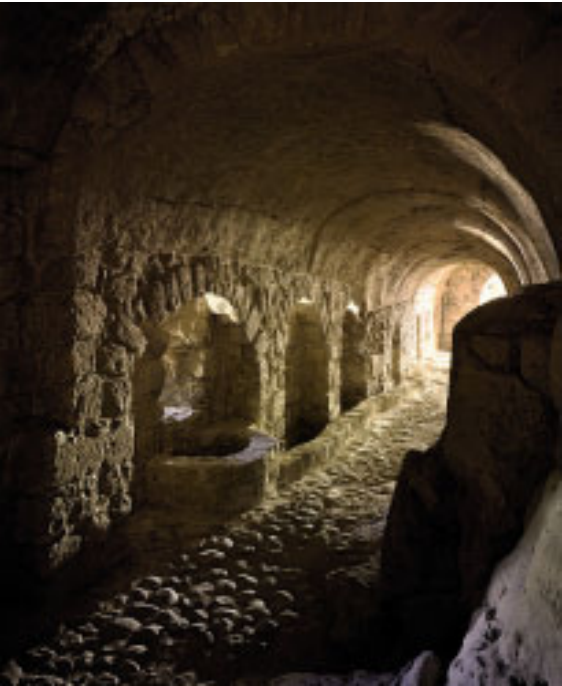
An access corridor in the Citadel is a 60-metre-long tunnel divided into sections separated by raised arches.
