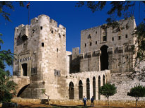
The bridge leads to the entrance complex.
