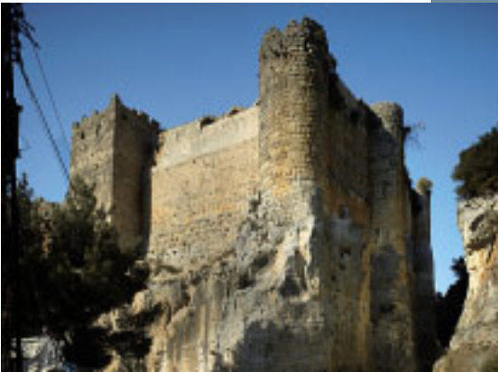
This view of the Castle reveals its Frankish fortifications resting on top of cut bedrock, with the rectangular tower and the moat in the foreground.
