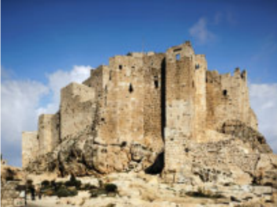
The facade of the Citadel of Masyaf, seen from the south, after several modern houses that had encroached on it have been removed.
