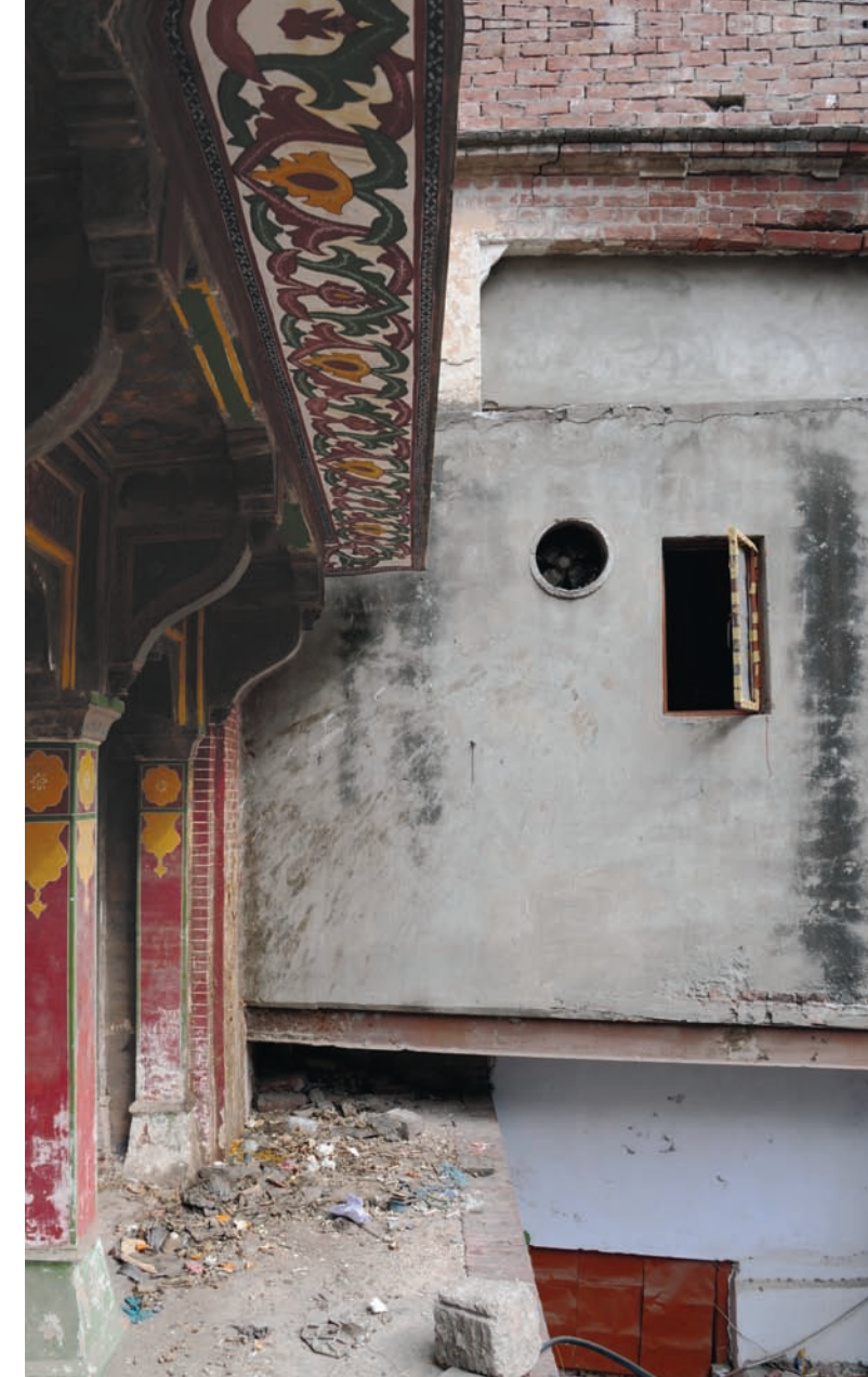
Opposite: A house abutting the south-western corner of the Calligraphers' Bazaar. It is impossible to ascertain where the original boundary of the mosque was.
