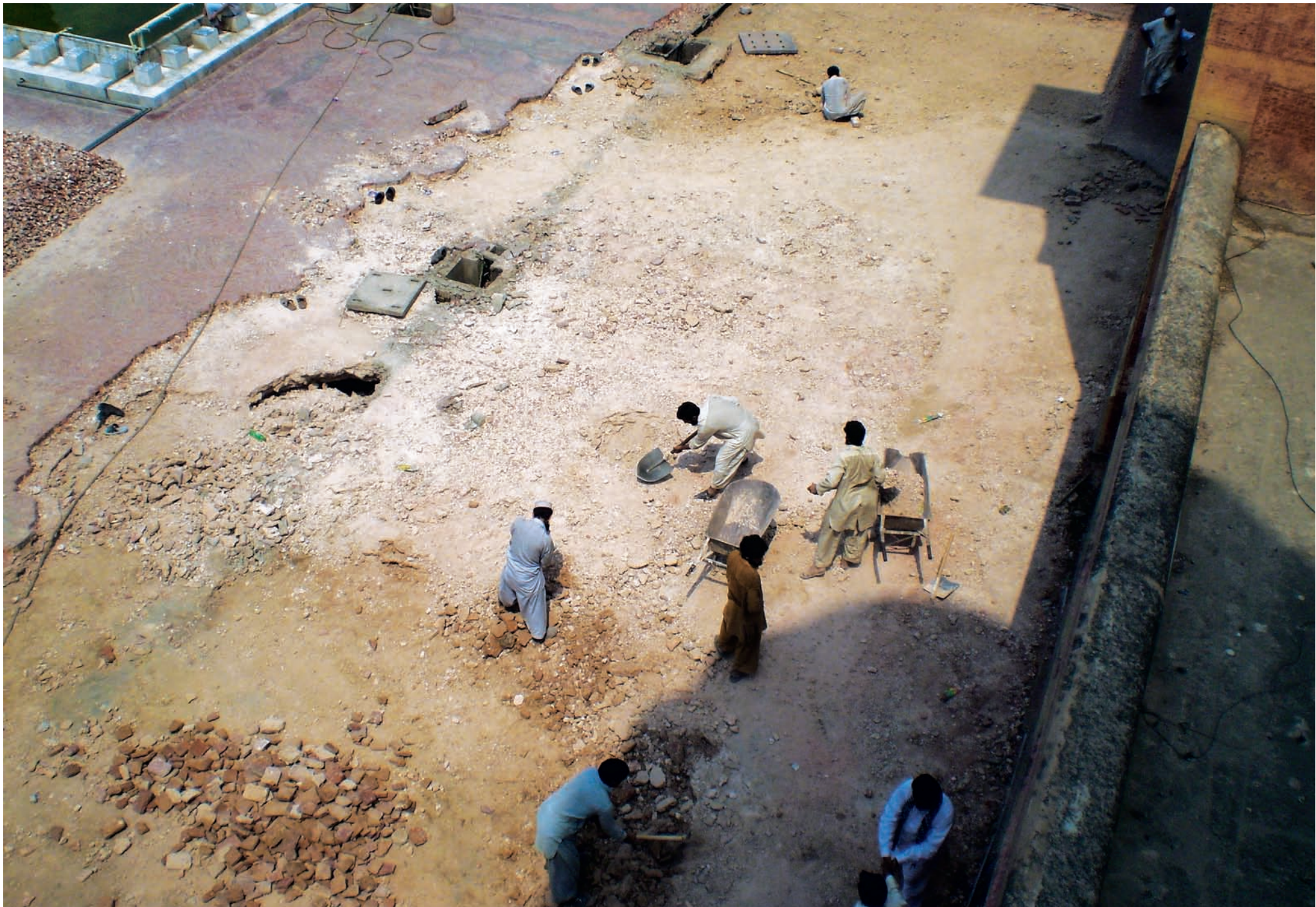
Close-up view of the excavation work.
