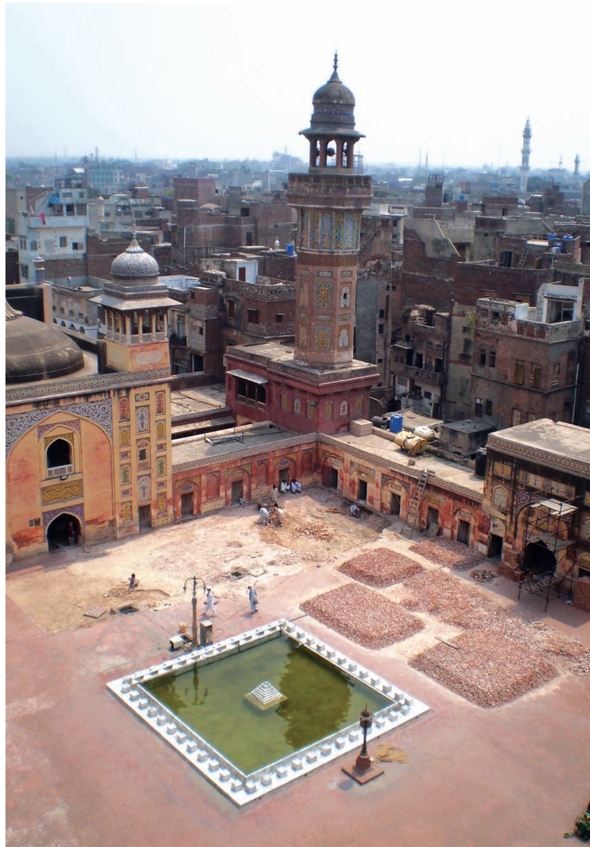
View from the north-west minar of the excavation work in the south-east corner of the courtyard.
