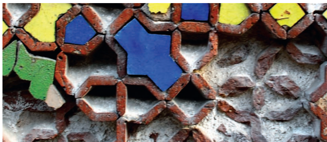
Breakout of tile embedded in unglazed terracotta lattice.
