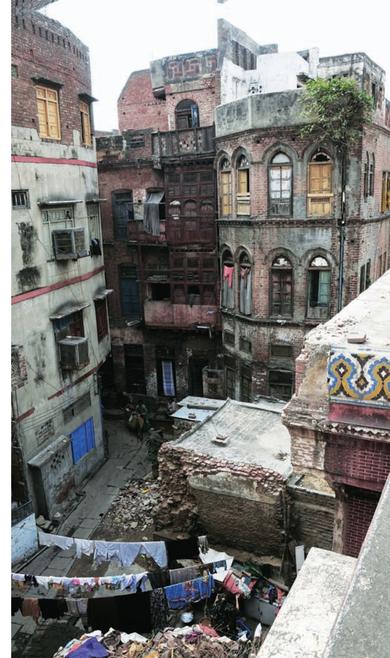
Above: View of the southern residential neighbourhood from the roof of the Calligraphers' Bazaar. Housing quality is poor, and solid waste management is minimal. The 3-storeyed building to the right of the photograph is built on the footprint of the original Persian well which supplied water to the mosque through the southern pavilion.
