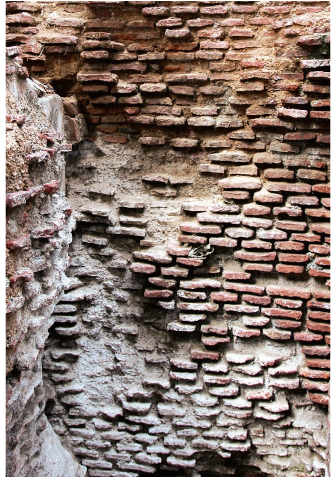
Sanding of mortar.
