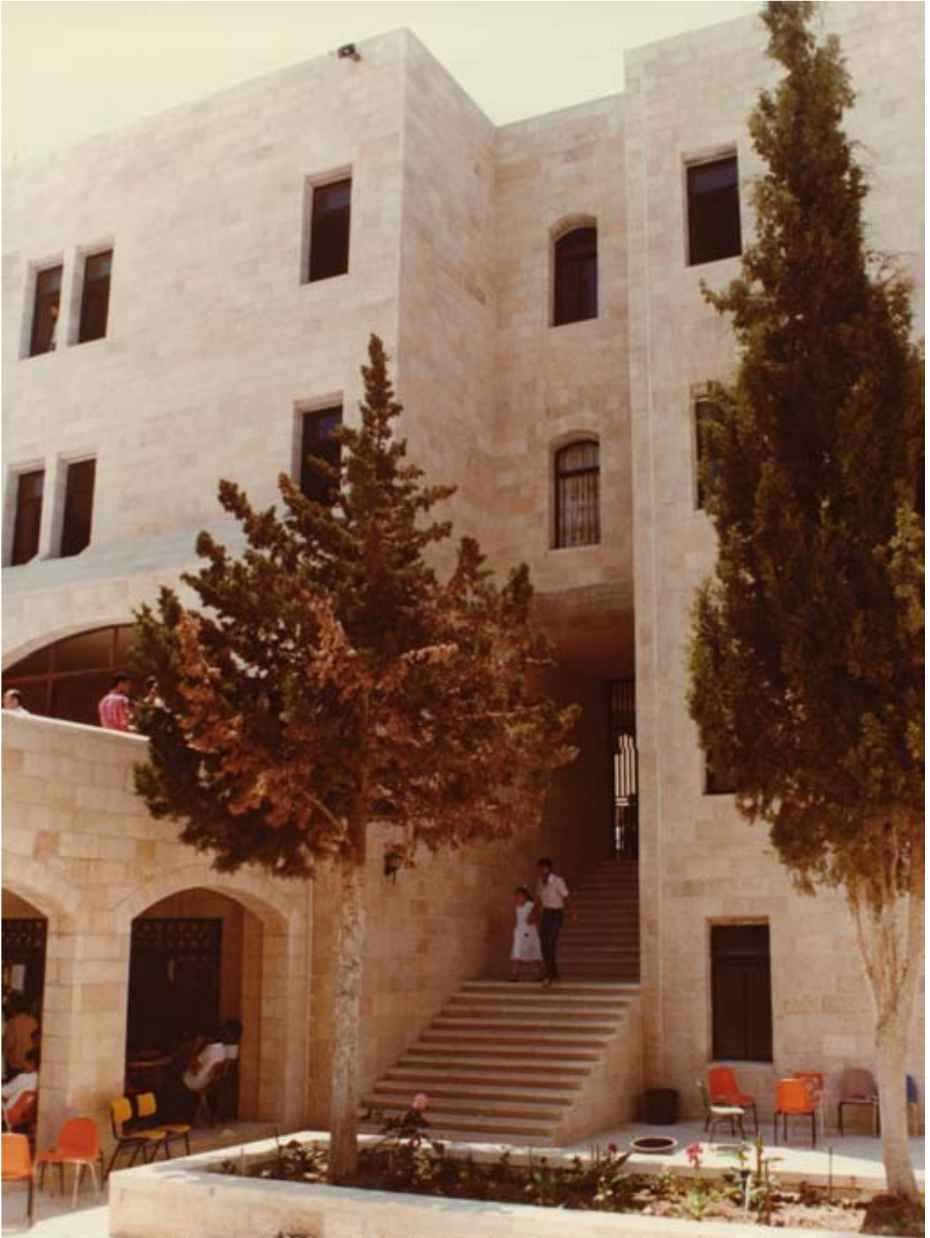
Connecting arcade and steps leading to west courtyard
