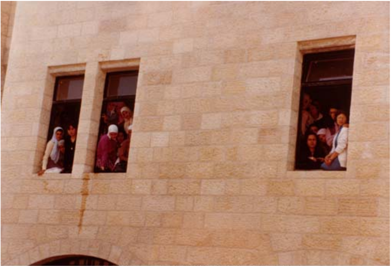
Rectangular windows in stone clad walls
