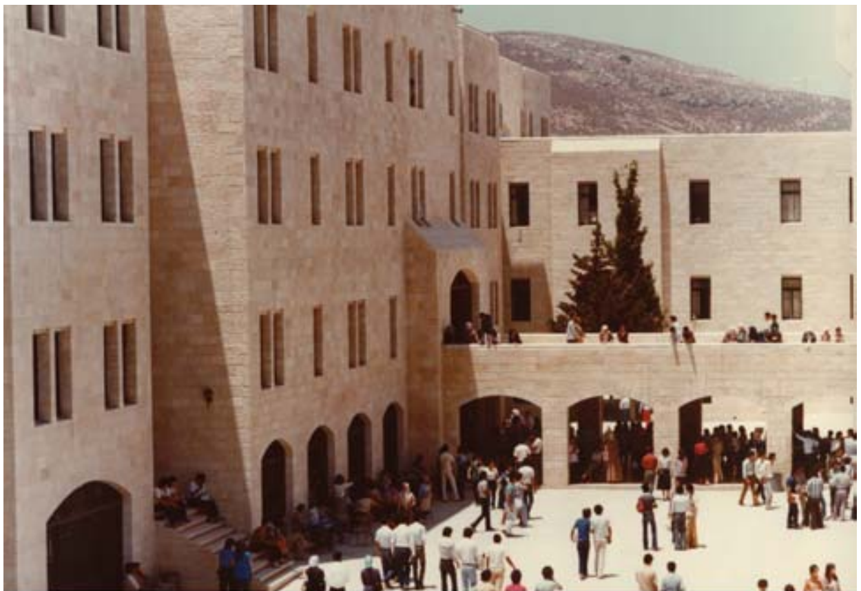
Northeastern elevation. The wing (right, background) and arcaded pathway connect annex to existing building (right)
