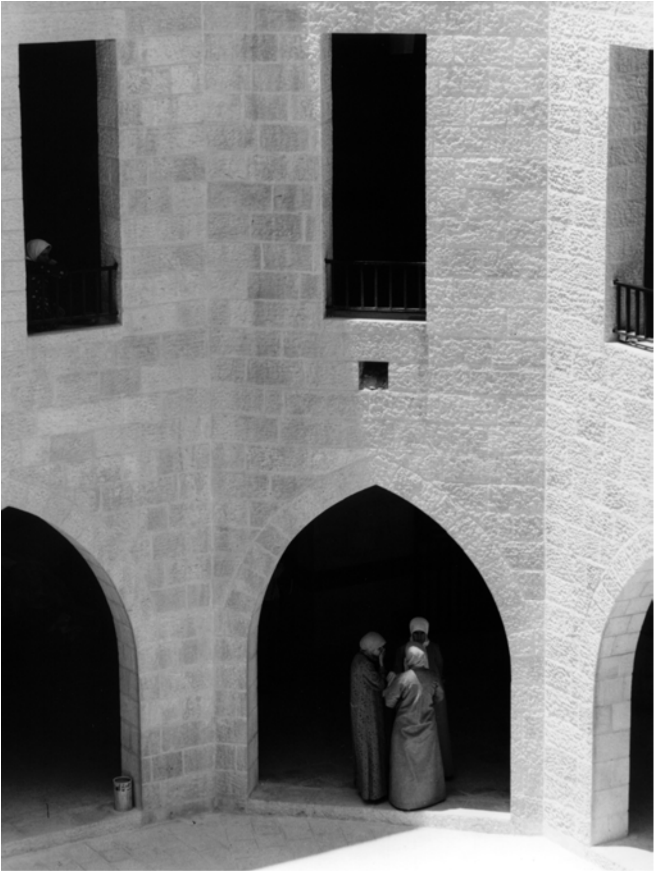
Detail of the corner of the east courtyard
