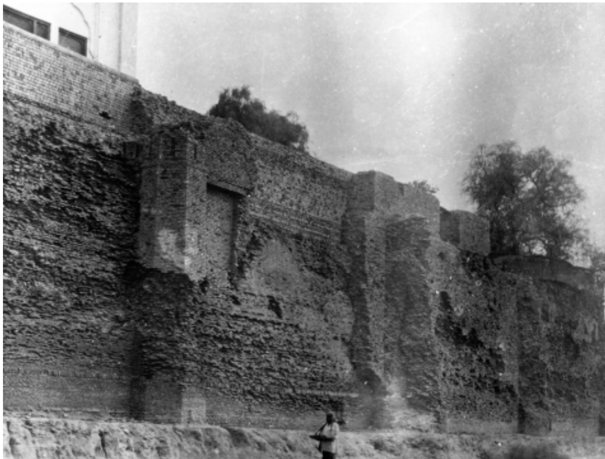
The high northern compound wall with exposed foundations exposed (before restoration)
