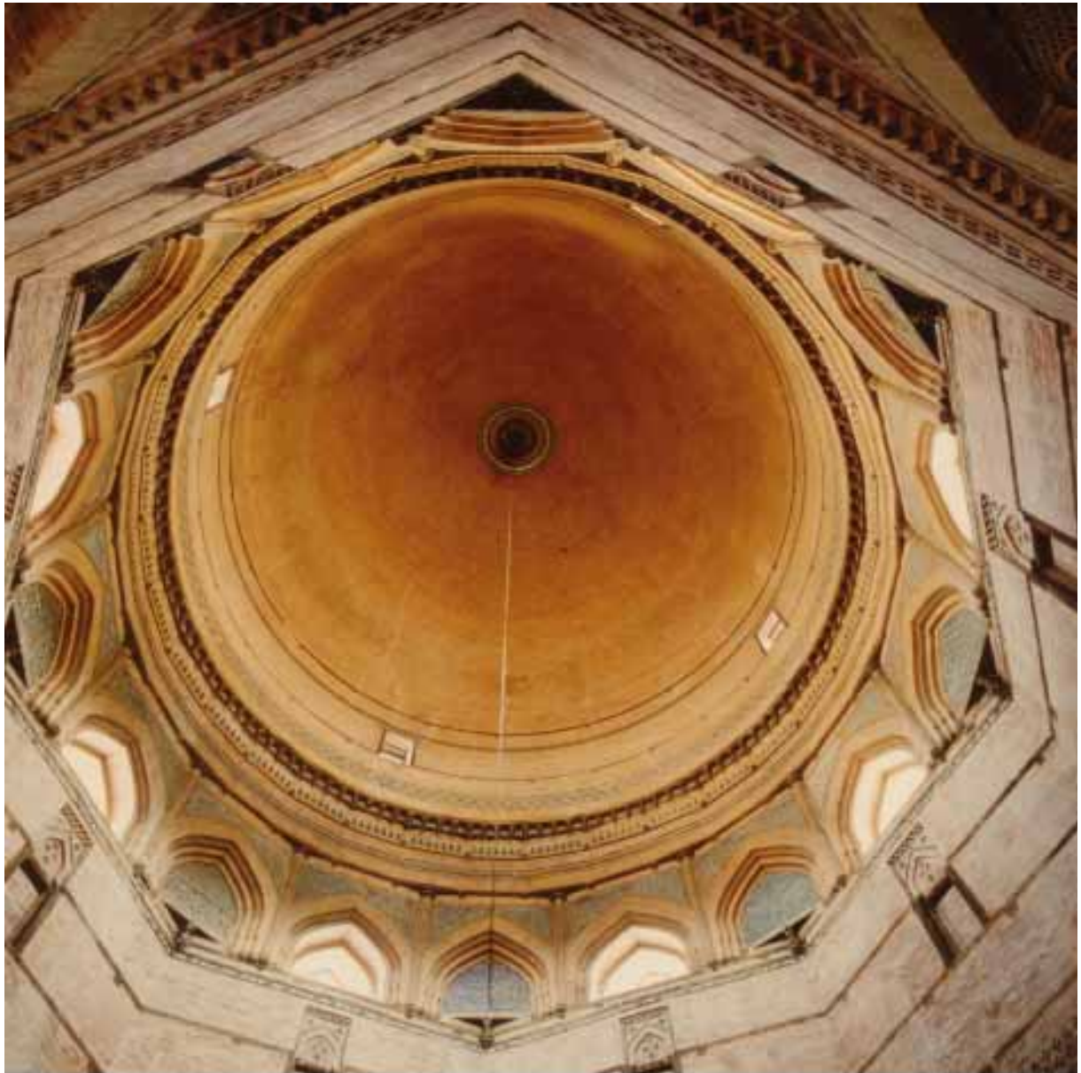
The interior of the dome and the drum. Note the repaired cracks in the dome
