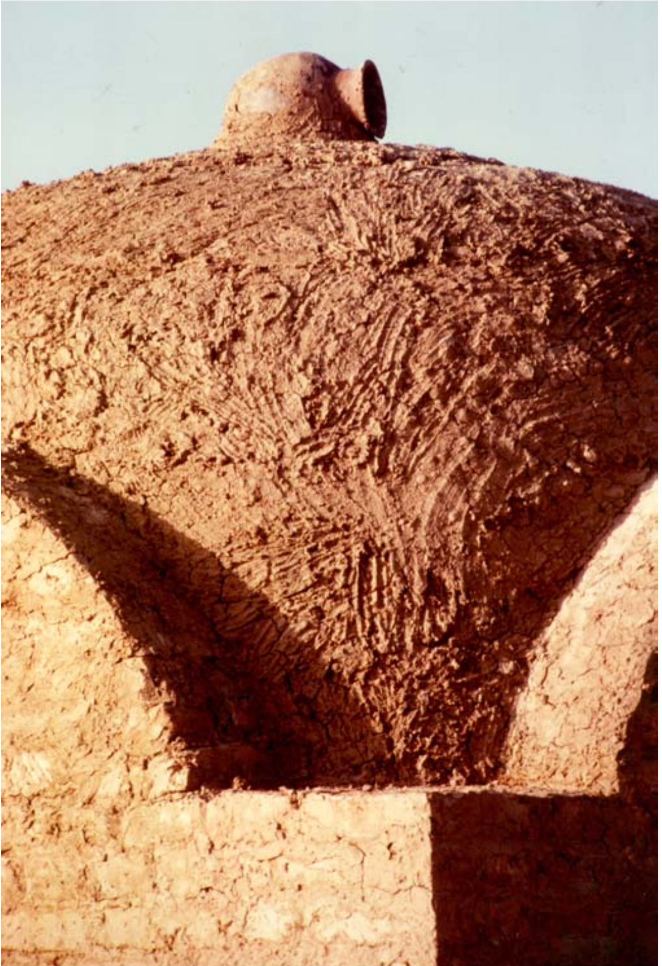
Prevailing winds pass over vase to draw off hot air
