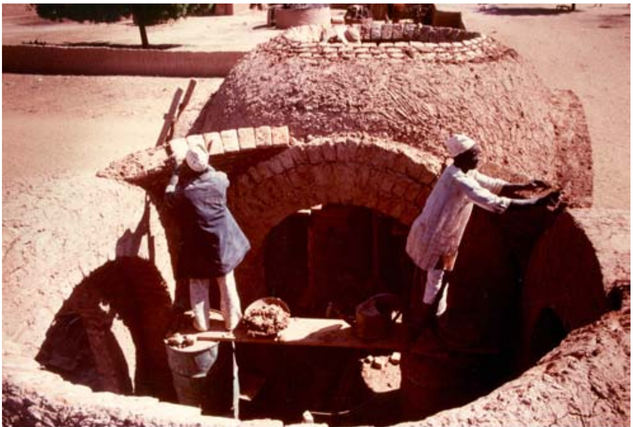
Interior and exterior surfaces rendered in mud with crushed accacia podes to increase water resistance
