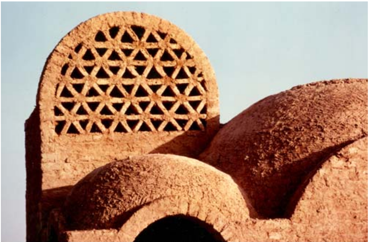
Claustra of wind-catcher; incoming air is pulled downward and passes of large ceramic jars filled with water
