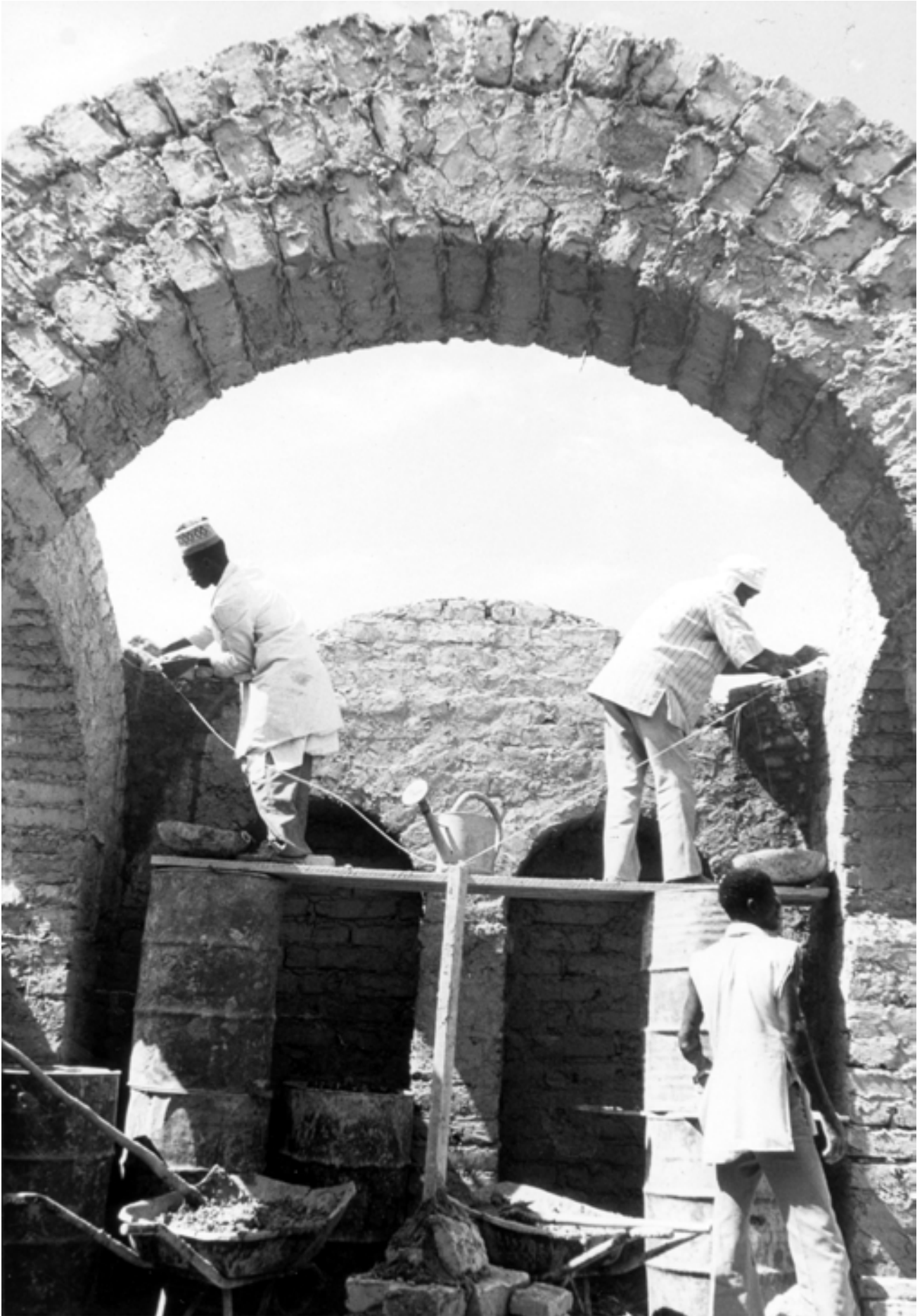
Construction of classroom dome: no timber shuttering used in Nubian/Iranian construction techniques
