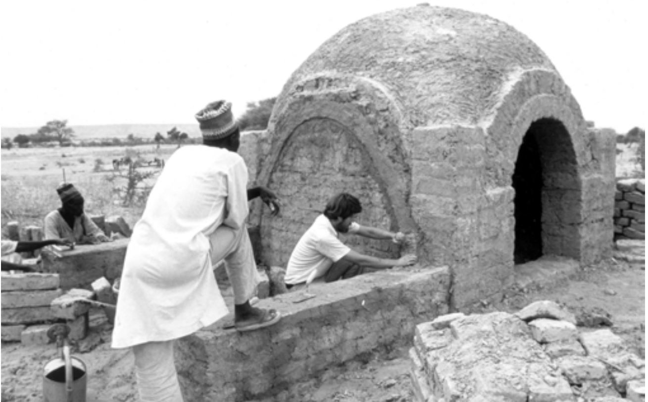
Local masons were trained in vault and dome construction; also given experience in foundations, walls, details
