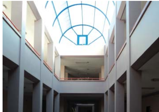
Figure 4: View from the Interior corridors-2 (Source: Authors, 2010).
