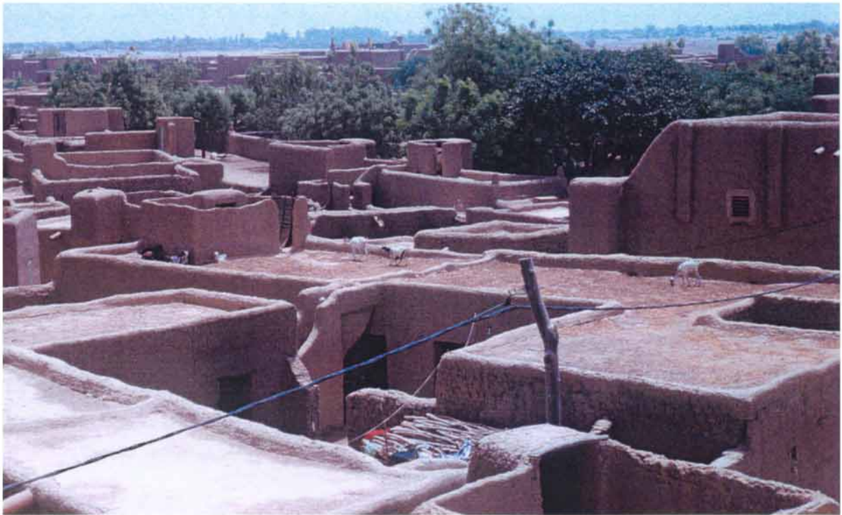
Above: General view over the flat mud roofs and courtyards of private residences.
