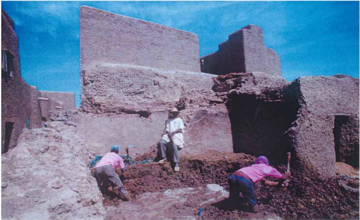
Above: Workmen mixing mud or banco dug from the floor bed of a site to be constructed. The mud will eventually be mixed with rice or barley straw before being shaped into bricks.
