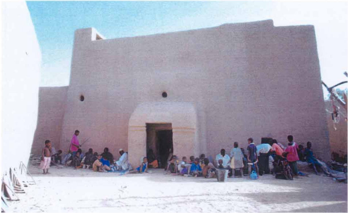
Above: Students gather in front of a recently rendered two-storey school. Minimal openings on the façade help keep the building interiors cool.
