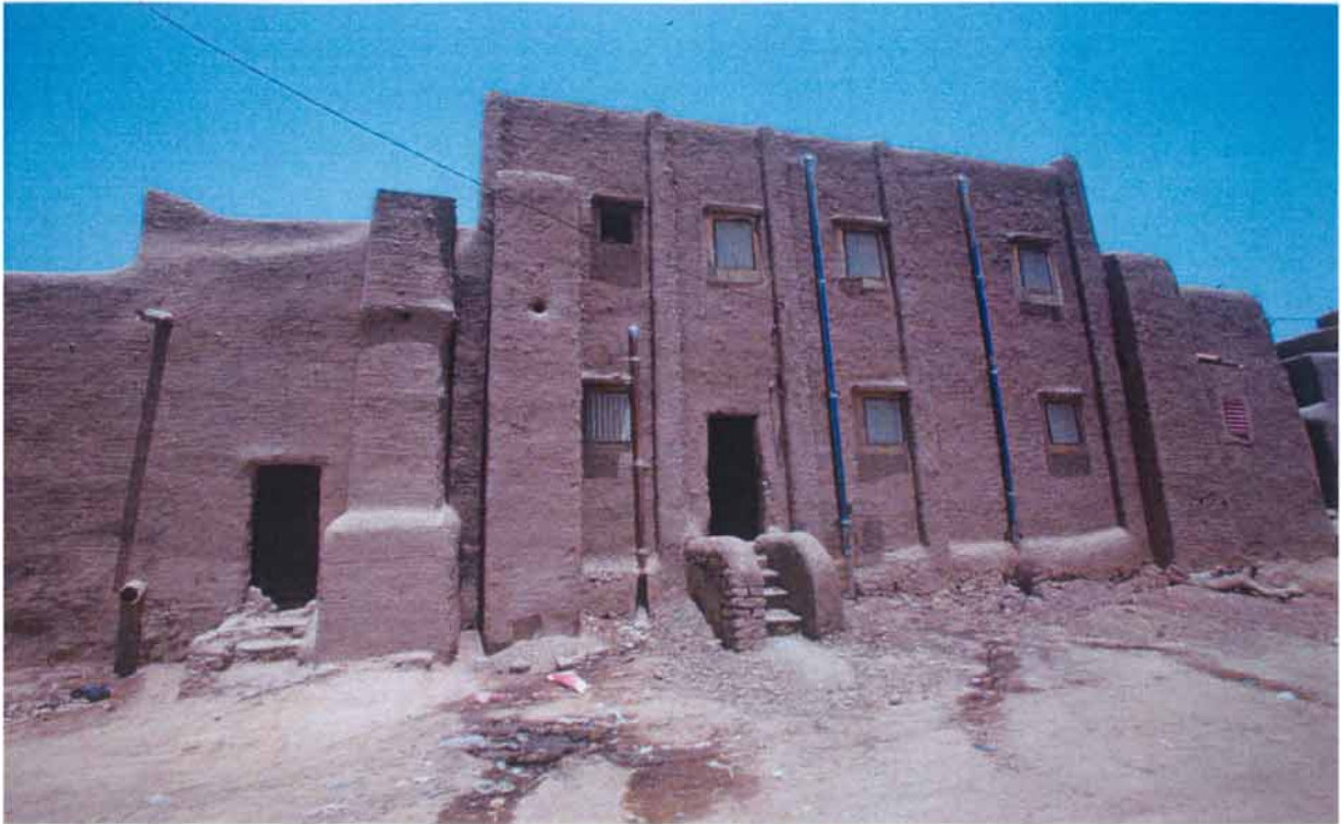
Above: The Moroccan style identifies this house as one of two-storeys containing an interior courtyard and belonging to an important family.
