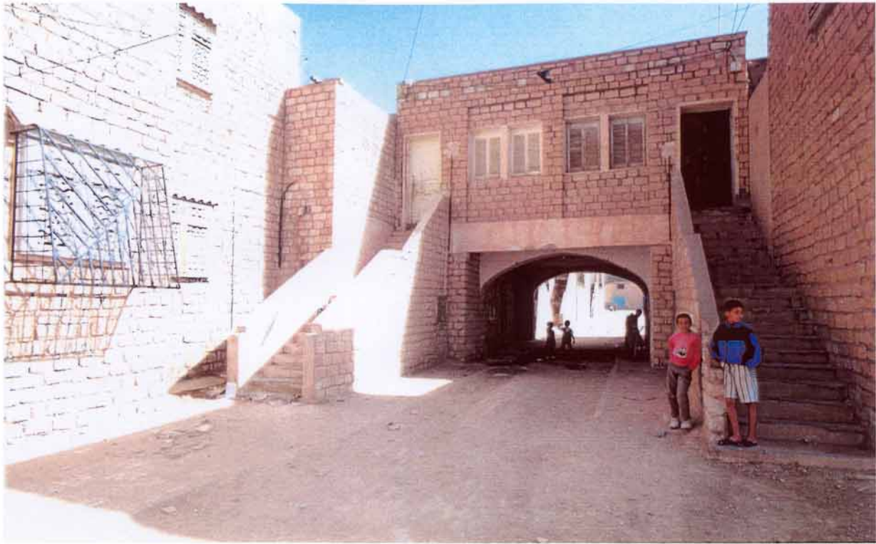
Above: Lime-sand stone extracted locally was used for the construction of the load-bearing walls. Floors, roofs and beams are made of reinforced concrete, as are the interior and exterior staircases.
