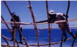
Two workers attaching poles with coconut ropes within the dome construction.
