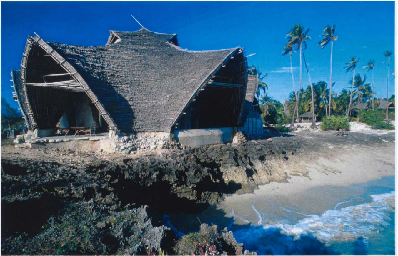
Above: Lattice-shell structures are built with kasuarinia-tree poles for the main struts and mangrove poles for the beams, joined with coconut ropes.
