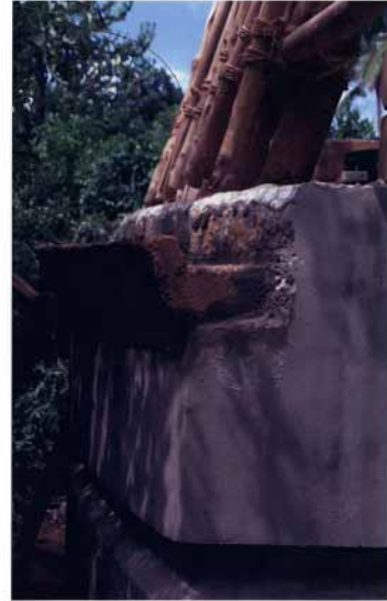
The rain water gutter below the roofing points of the roof frame is wide enough to collect tropical rain. The groove running around the base of the bungalow is a measure to prevent termites from entering the house.
