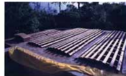
The joints between the sand-cement blocks, placed on the formwork, will be filled with concrete. Once the concrete is hardened, the formwork will be removed from the cistern chamber through the revision hatch.
