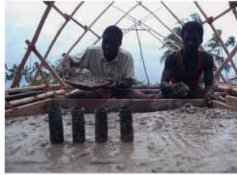
Two workers concrete the platform inside the 'technique tower' which will eventually carry the hot water tank.
