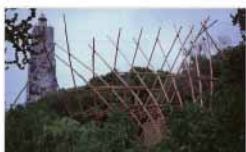
The upright frames are propped up by temporary supporting poles, until ...
