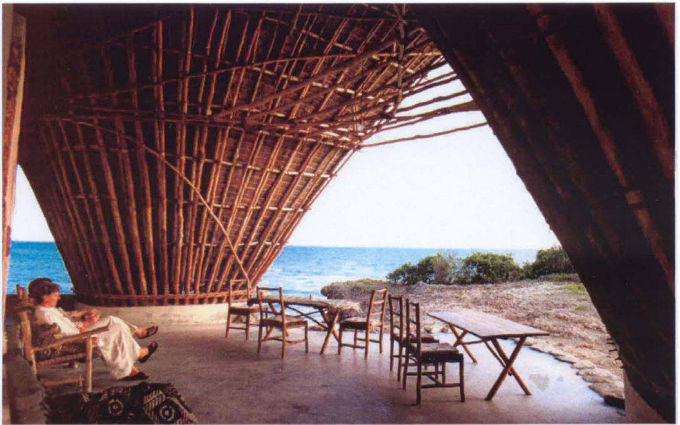
Above: The wood lattice structure covers a wide area with only few points of anchorage, allowing open views and natural ventilation.
