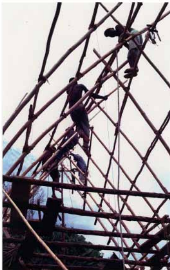
Workers attaching the ridge to the upright frames.
