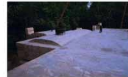
Standard plastic tubes and bucheles are used to make openings for water pipes and the compost toilet refuse opening in the vault.
