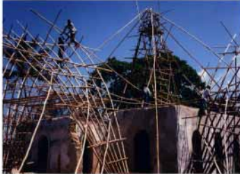
For the construction of the free spanning roof dome of the Visitors' Centre, six lashed shell modules are built simultaneously to meet in the centre of the construction, forming its vertex.
