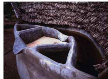
A filter and four foot unit in use. According to the prevailing water level, the water flows into the next partition.
