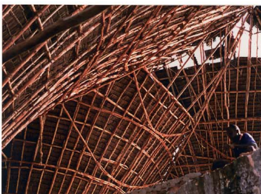
Part of the 21 m free-spanning roof construction, built from slender local poles
