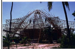
Dome of the Visitors' Centre under construction is probably the largest free-spanning dome made from slender poles and coconut ropes.
