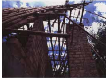
In contrast to the solid 'technique tower' and the partition wall to the bathroom, which are made from blocks, the light roof is made from local poles.
