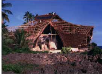
The roof dome is partly covered with mauuli. Solar panels are installed to provide energy for lighting and radio communication to Zanzibar.
