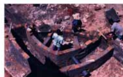
A filter and four foot unit, which also forms a footing point of the roof dome.
