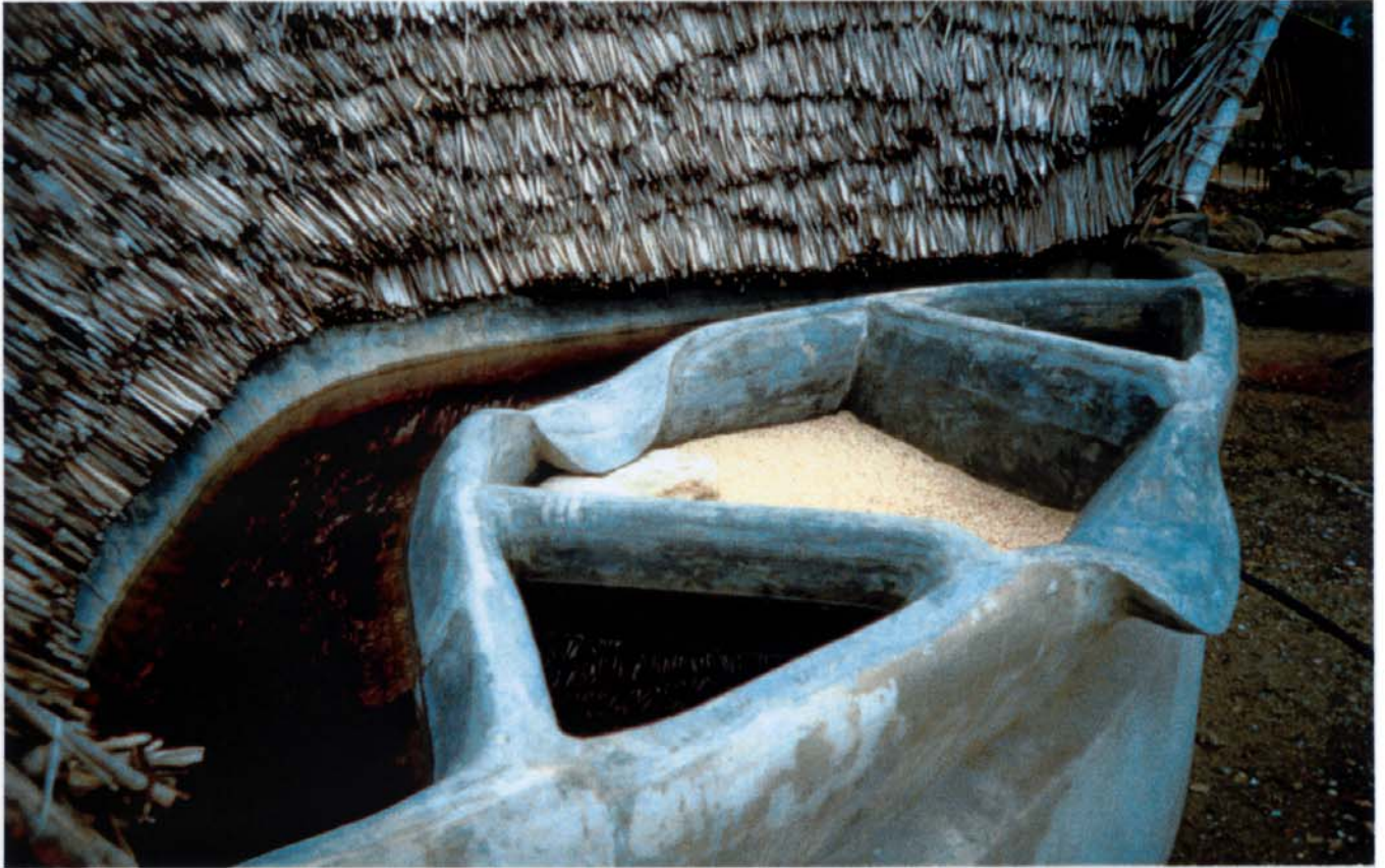
Above: Rainwater filter and flush basin in the Visitor's Centre.
