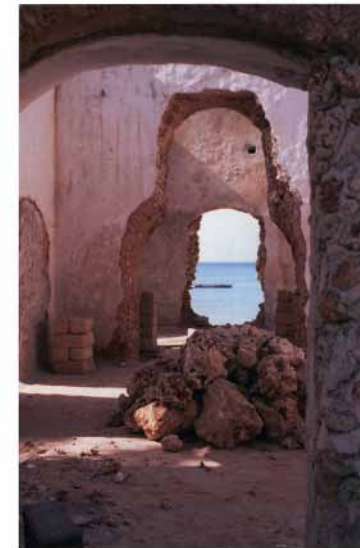
Much of the doors and windows of the lighthouse keeper's house are widened and enlarged.
