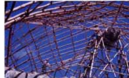
Finally the six modules join up in the centre, forming the vertex.
