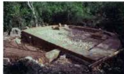
The foundation of the cistern is ready to be filled with concrete. The compost chamber is shaded with coconut palm leaves to ensure curing of the plaster.
