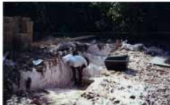
The compost chamber has been excavated from the coral rag. The first blocks of the chamber are laid by Abd. the foreman.
