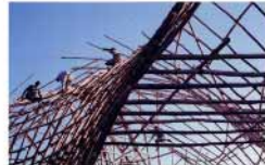
One lashed shell module under construction.
