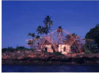
The bare pole construction of the roof dome spans over the former lighthouse keeper's house.
