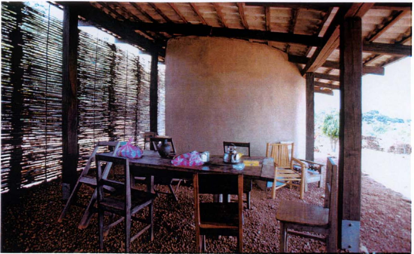
Above: The floor in the open spaces between the rooms is covered with red laterite gravel.
