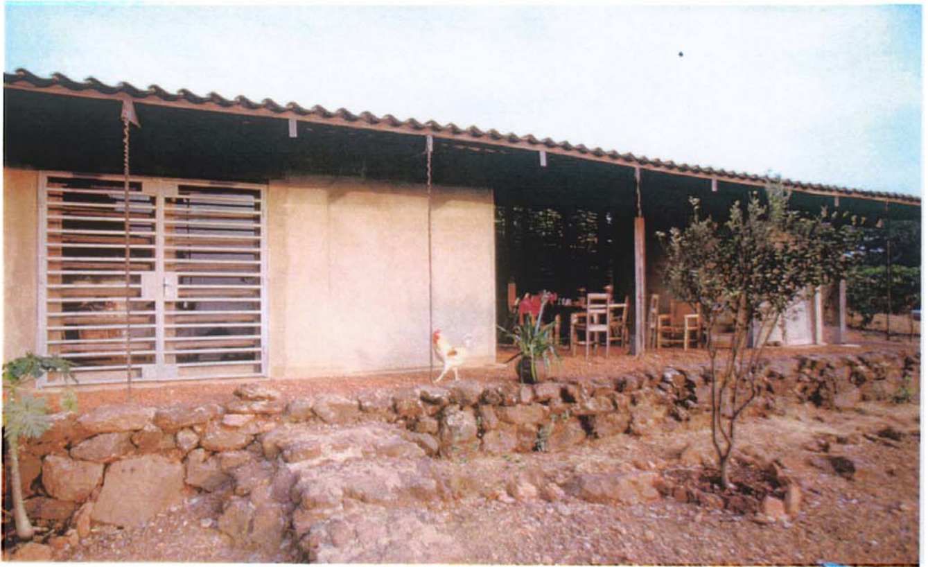
Above: Vertical cables tie the roof down in case of high winds.
