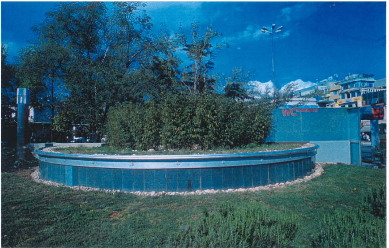
Above: The circular structure containing the washroom facilities protrudes 1.1m above the ground and is surrounded by opaque glass allowing natural light to penetrate the interior.
