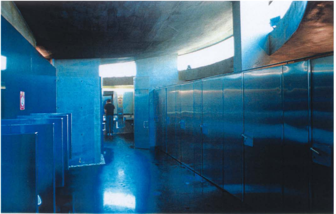
Above: The interior of the men's washroom is detailed in stainless steel and granite floors. The structure is a concrete shell.
