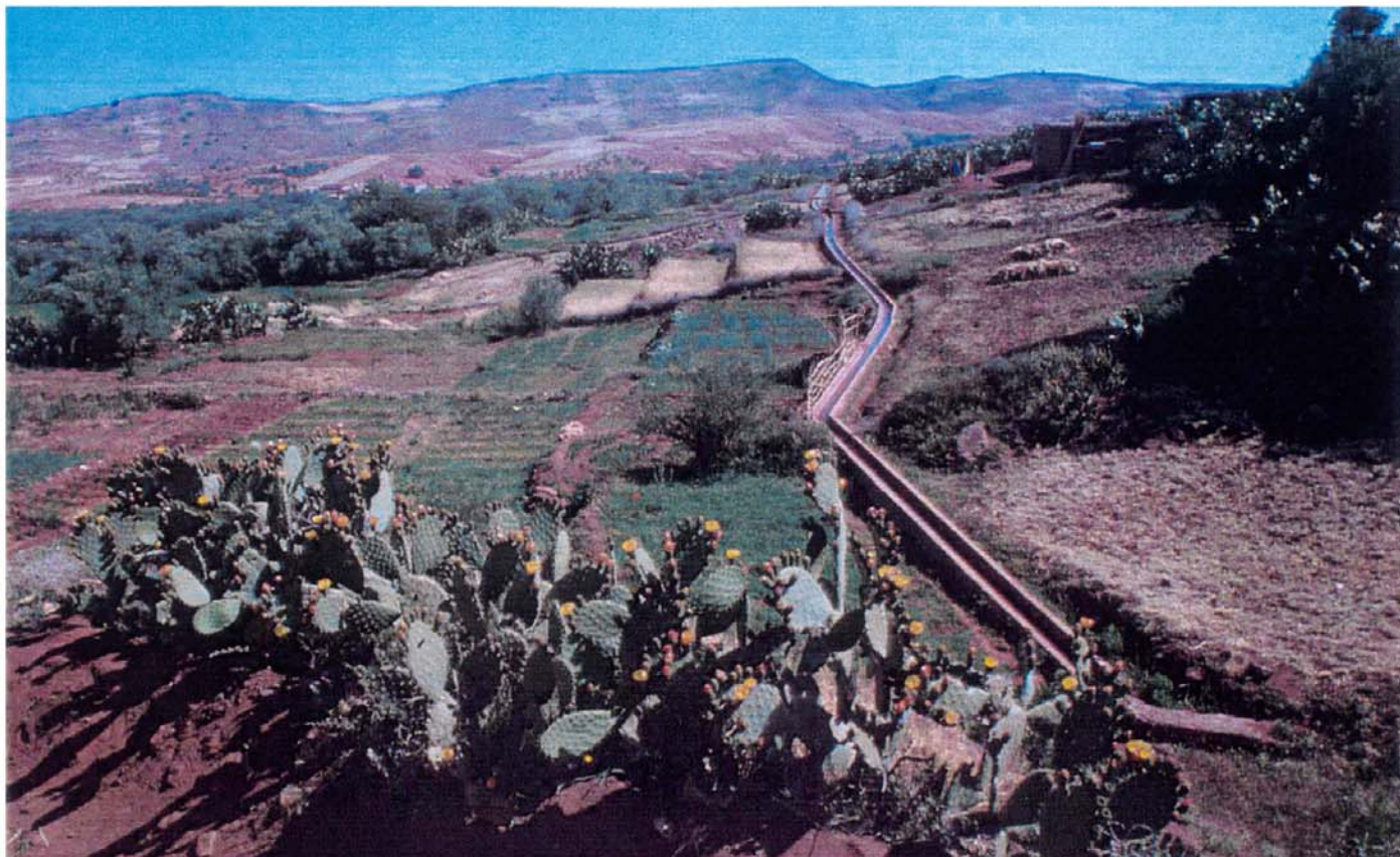
Above: A new canal, 2.5 kilometres in length, has been built in reinforced concrete on the location of a former earth channel east of the village.
