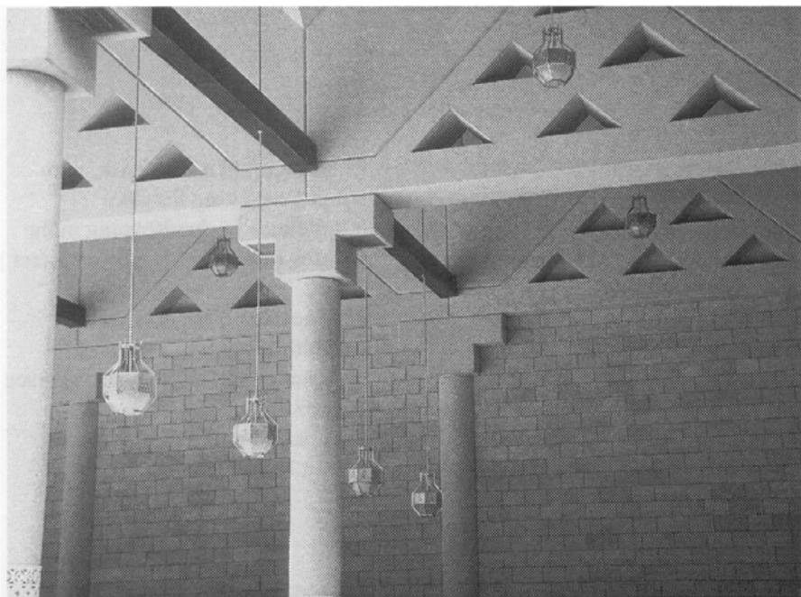
Detail of structural column and beam
