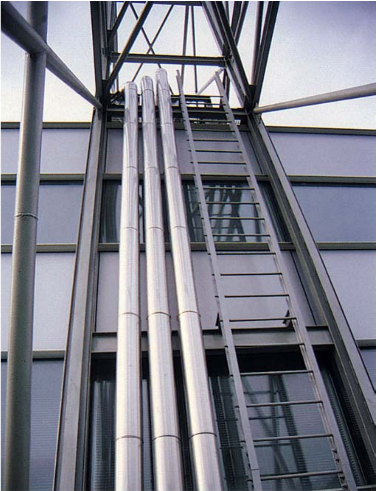
Yalova-Elyaf administrative annex This double-sided board also provides room for the mechanical systems that extend from the ground to the roof
