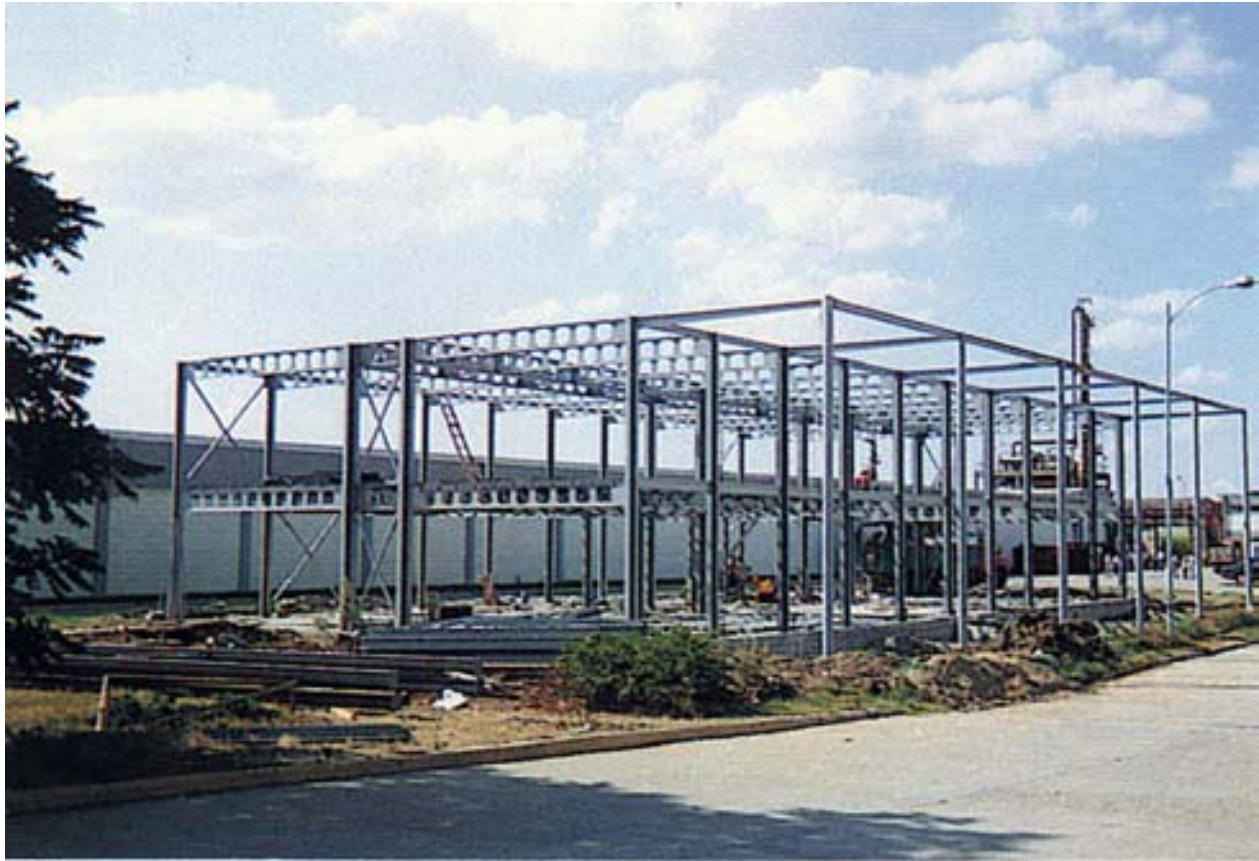
Yalova-Elyaf administrative annex Phases of the steel construction process
