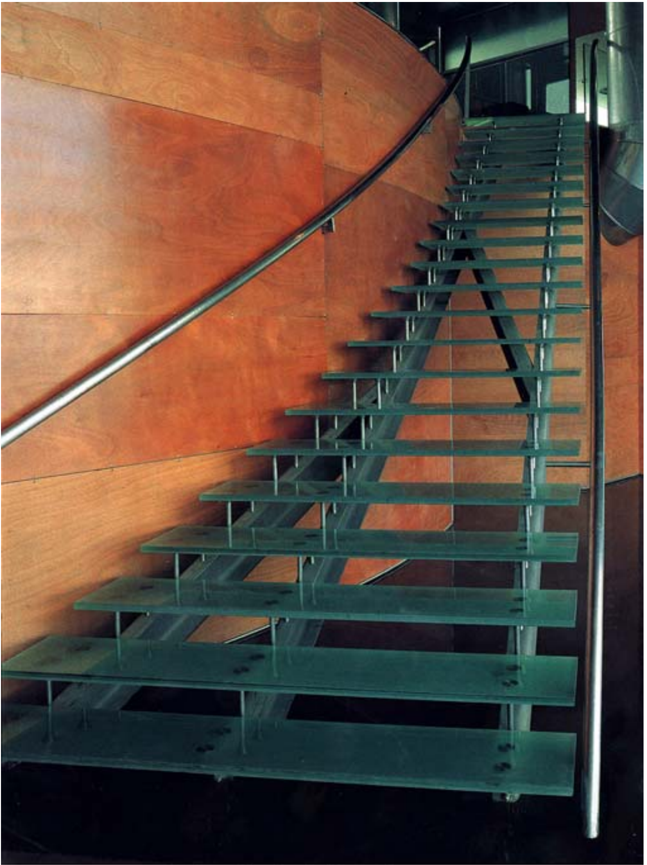
Yalova-Elyaf administrative annex The staircase consists of laminated glass steps (3x10mm thick) fixed onto a steel structure. Two asymmetrical steel handrails appear on both sides of it
