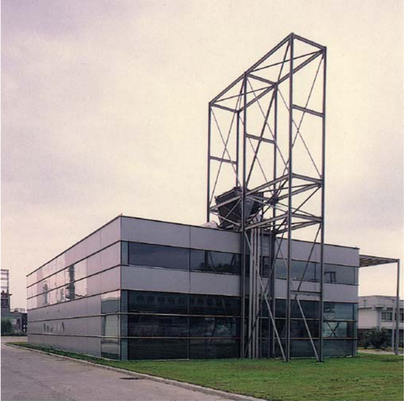
Yalova-Elyaf administrative annex The steel structure attached to the south facade will serve as a support for the factory logo board
