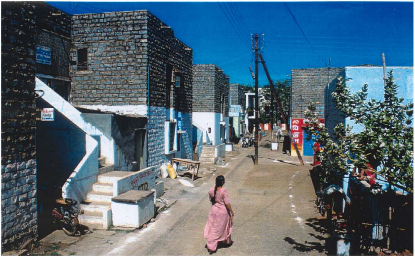
Above: An important element of the overall design is the way that everything – from the pathways to each component of the units – is built from stone, giving a feeling of homogeneity to the whole project. The use of rubble stone walls gives a low-maintenance external finish.
