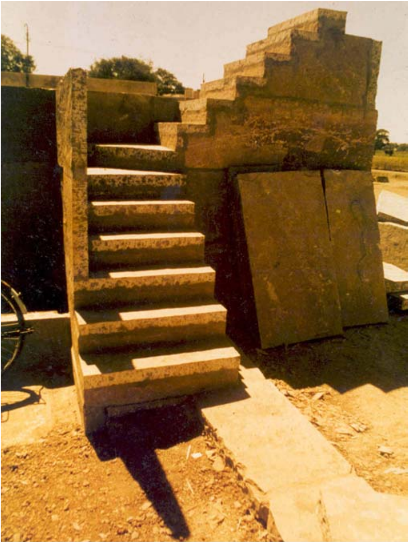
Method of construction showing erection of staircase with stone slabs and supporting walls,parapet etc.,by dovetailling slabs on edge with the help of iron clamps
