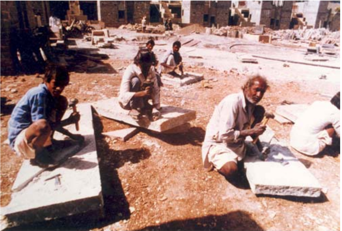
Preparation and dressing of various building components by manual labour on site
