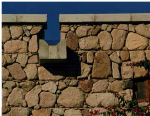
RAINWATER SPOUT DETAIL
