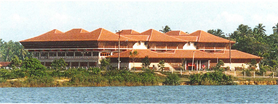
1. Artist's retreat, Diyabubula, Dambulla (1989). The upper platform is used for sleeping, whereas the dining area, pantry and a toilet are below. Bamboo tats along the perimeter keep out the wind and rain. (Photo: Laki Senanayake.)
