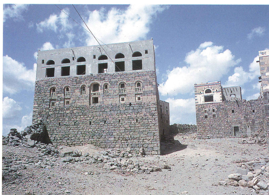
9 The town of Mangadah after the 1982 earthquake in the Yemen Arab Republic. Loss of traditional building skills, lack of maintenance and scarcity of timber were among the factors for building collapse.
