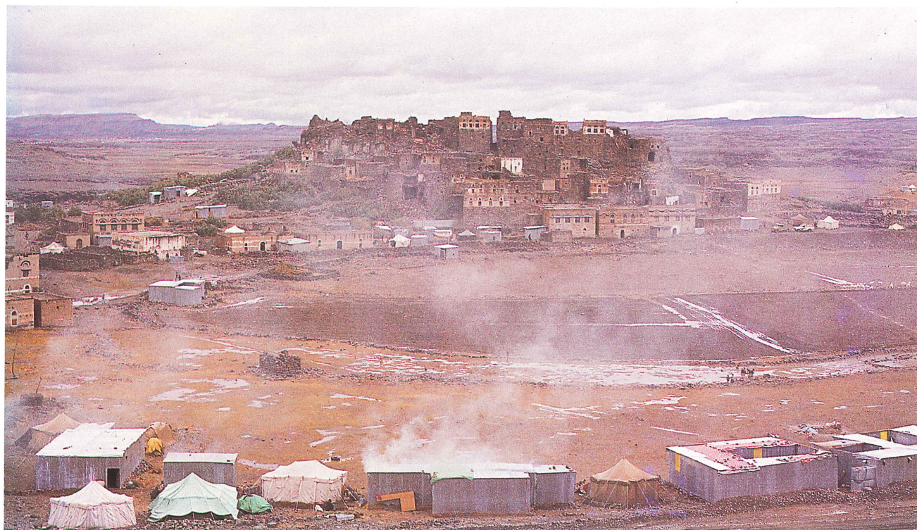
9 The town of Mangadah after the 1982 earthquake in the Yemen Arab Republic. Loss of traditional building skills, lack of maintenance and scarcity of timber were among the factors for building collapse.
