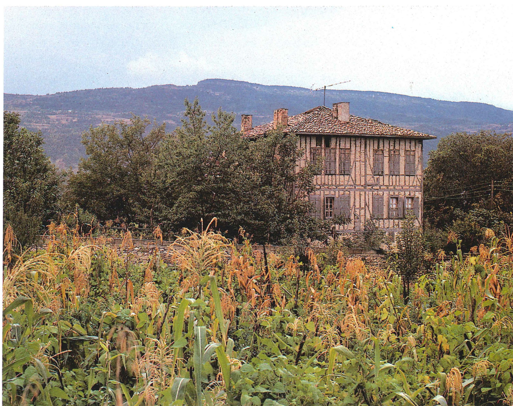
Left: Houses with tiled roofs in Yörük. Above: Four-storey house in Yörük. Right: Typical wooden framing for upper storeys, with mud brick or stone infill which is then given an outer coating as a rule.
