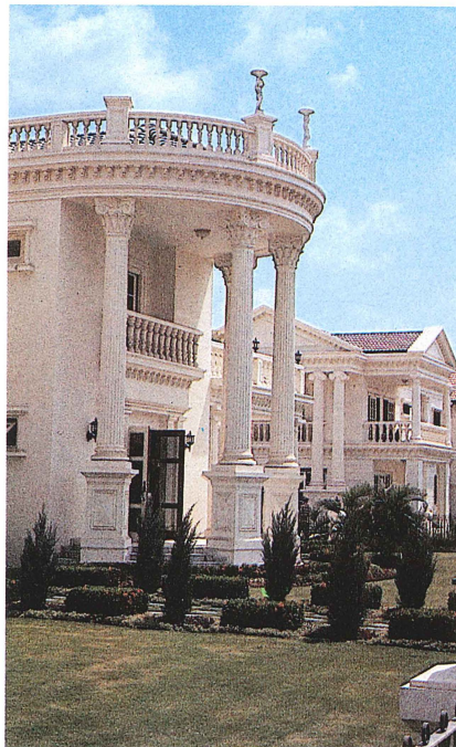
Sukhumvit Garden city in downtown Bangkok under construction. Housing in "Style Louis...". Photograph: Brian Taylor.
