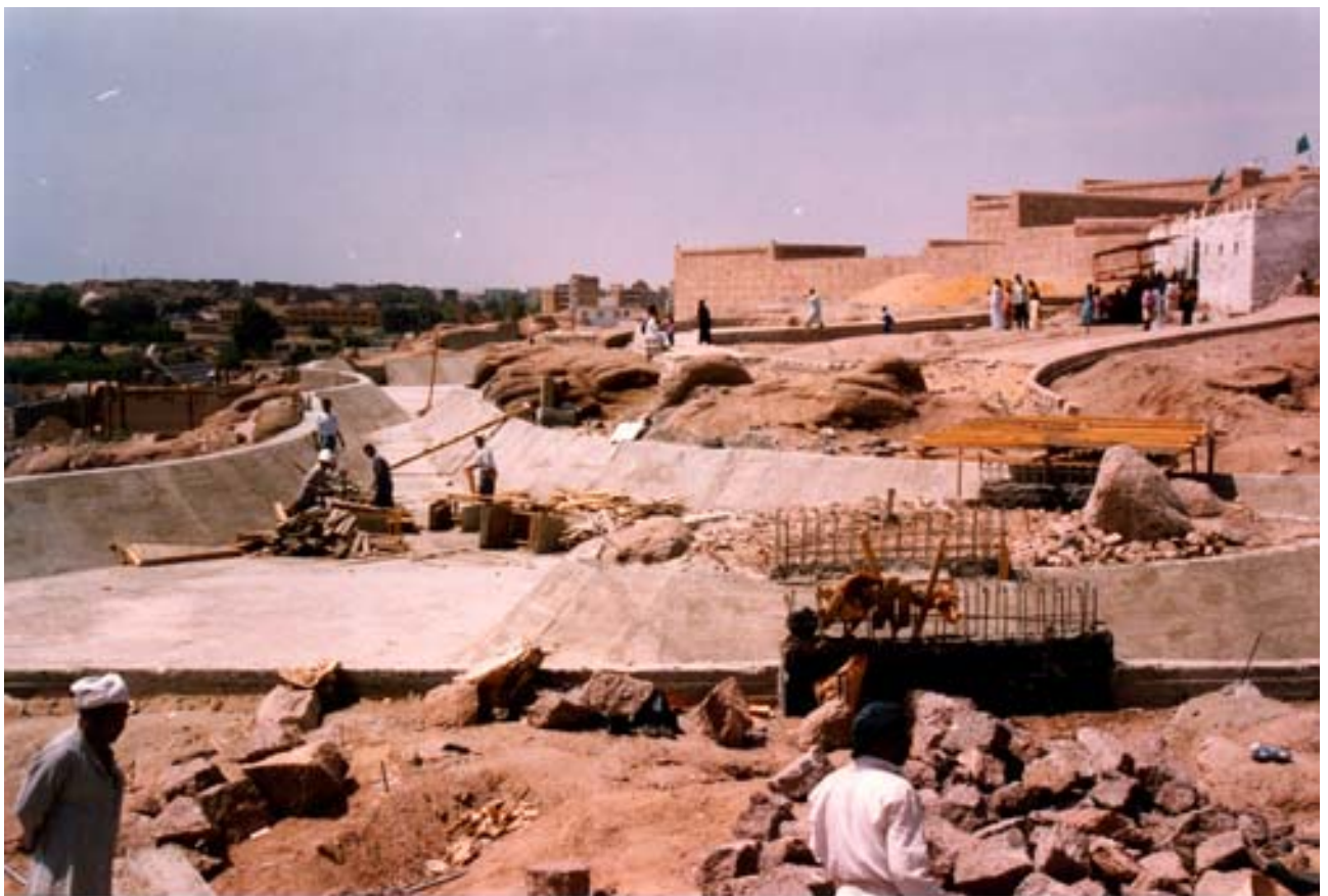
Retaining wall for the lack
