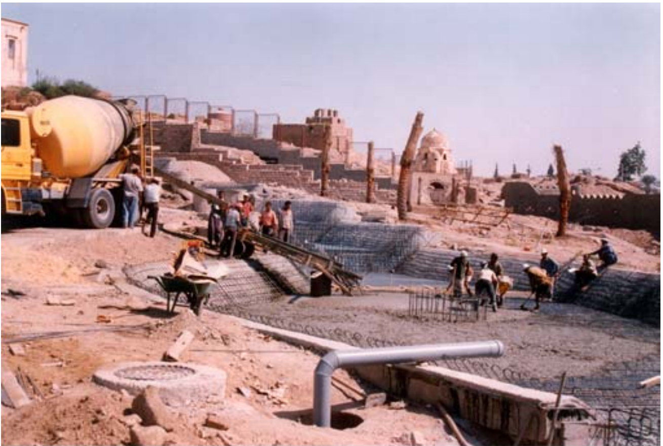
Steel reinforcement works at lack
