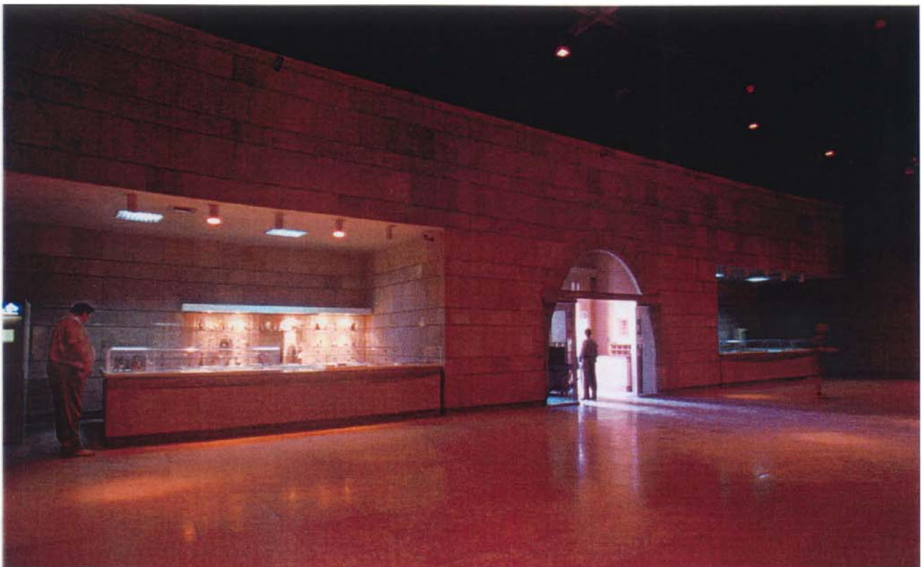
Above: The structural system of the museum is a reinforced-concrete frame with concrete block infill panels clad in sandstone. The design language refers to elements found in traditional Nubian architecture.
