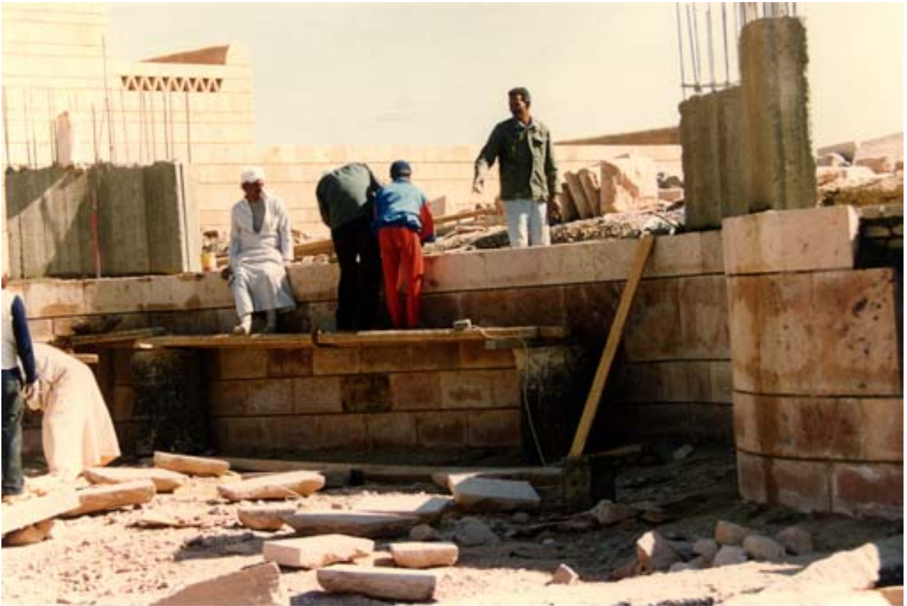
Retaining wall at front elevations
