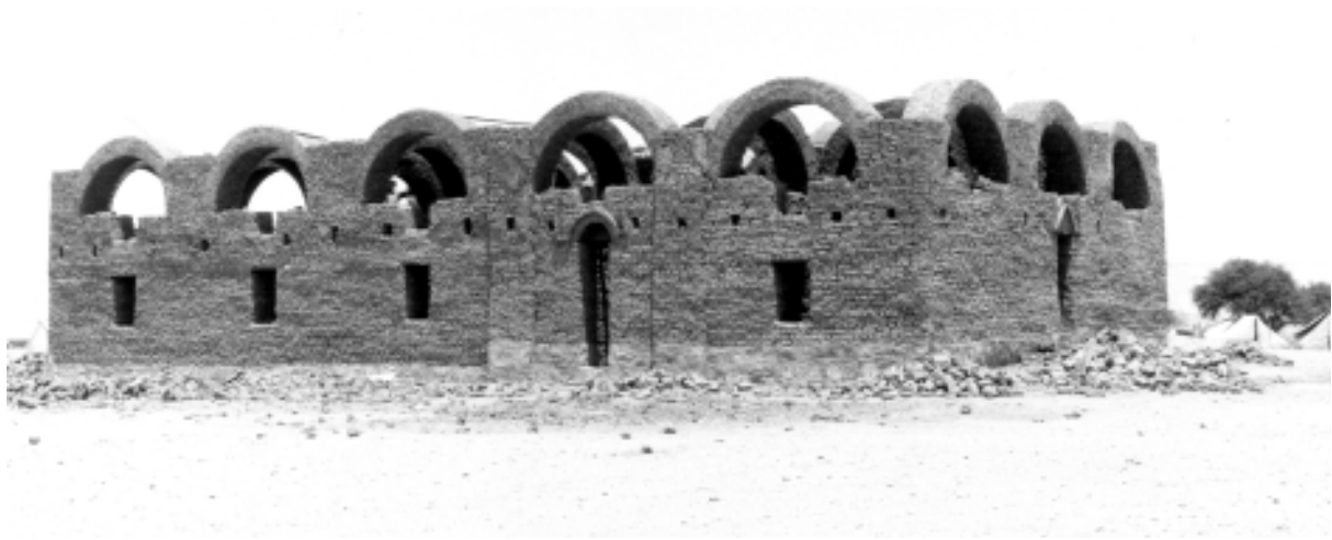
The main workshops (north wing) under construction.
