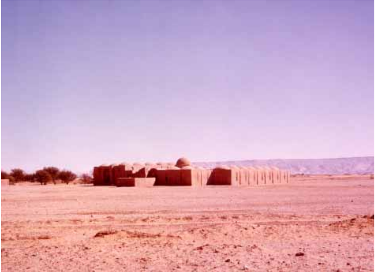
General view from SW: main workshops and store houses; 7 individual rooms
