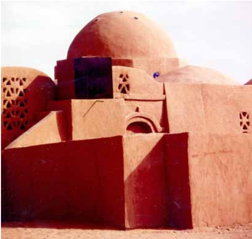
Exterior view of the kitchen yard (foreground, and stairs (centre); main dome of reception room
