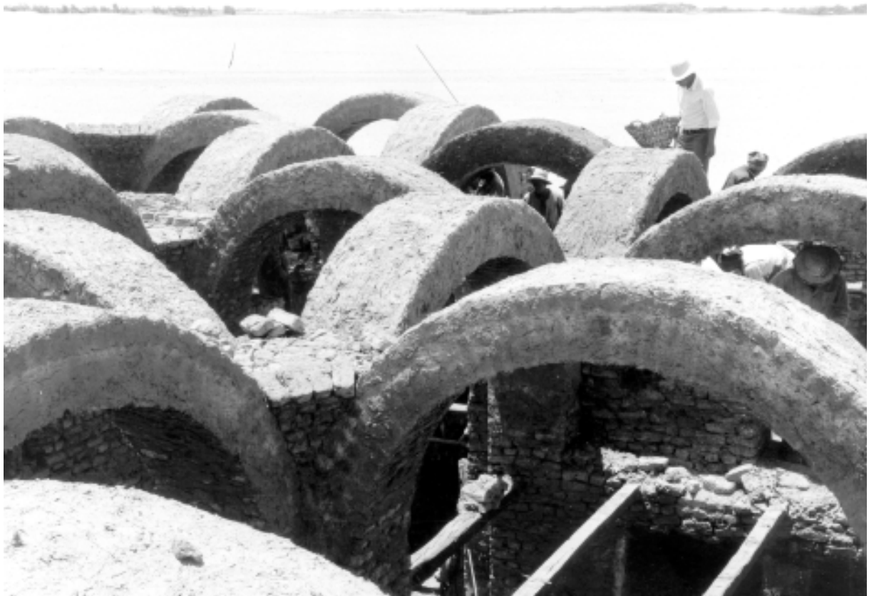
Detail of the arches before erection of domes.
