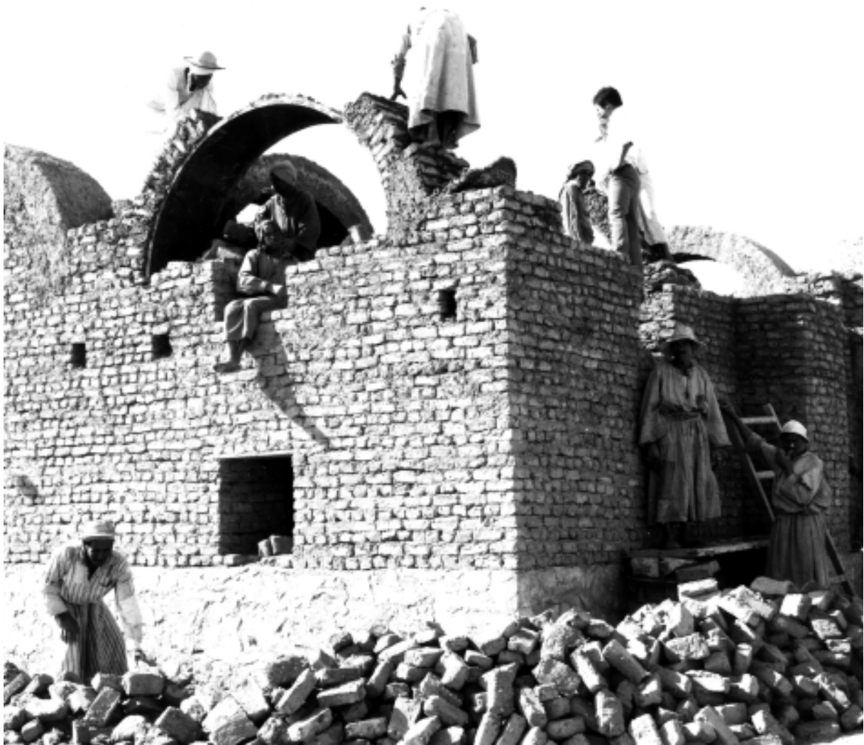
Arch construction in adobe bricks utilising a metal formwork.
