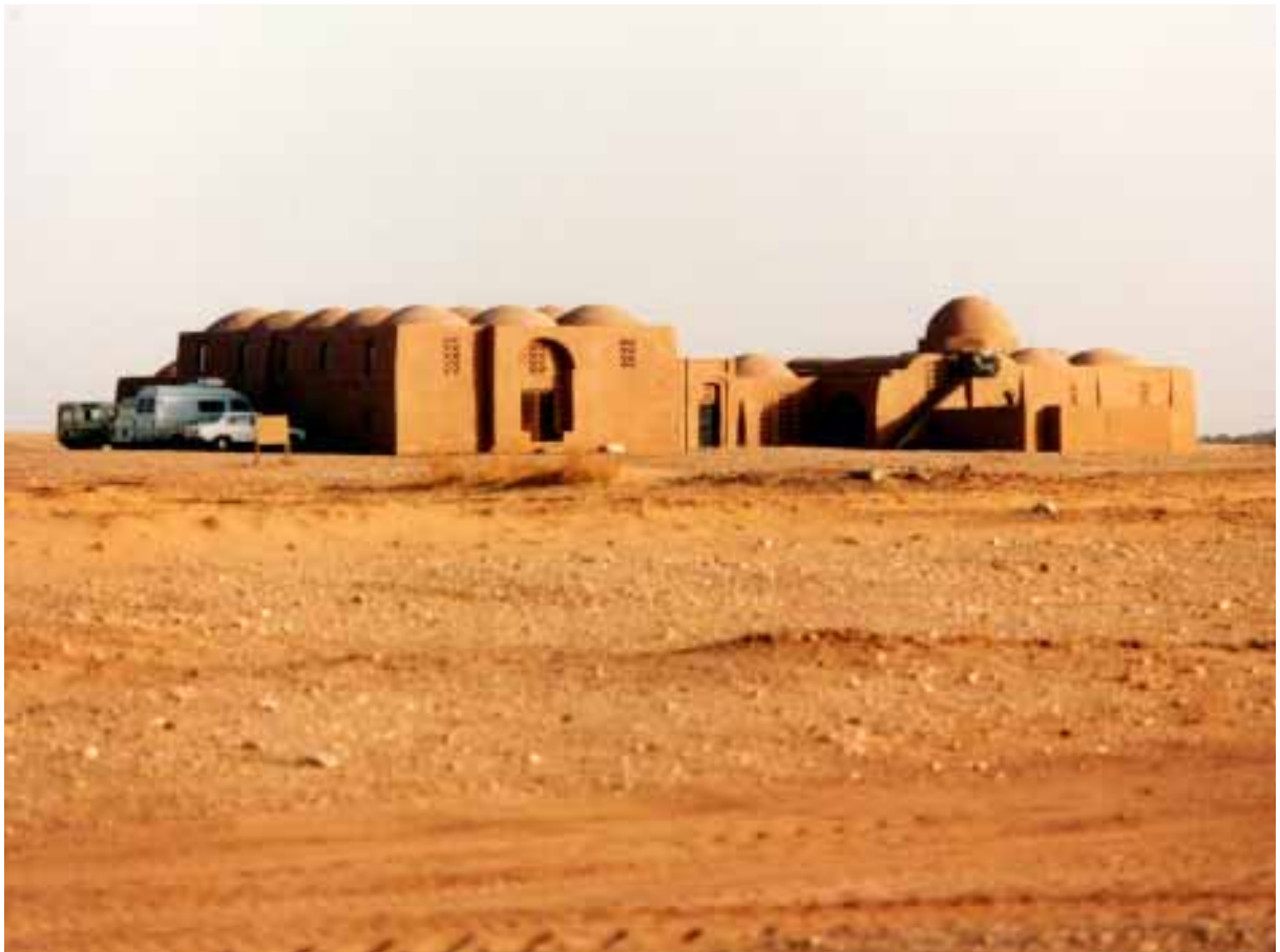
View from NW: main entrance (centre); access to workshops (left); roof (right)
