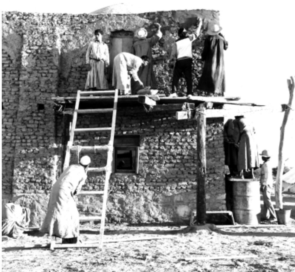
North wing under construction; plastering.
