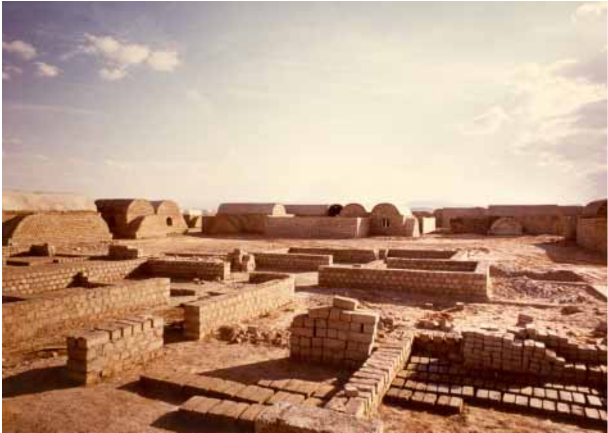
10 masons trained in construction techniques. Mud bricks stabilised with 6% concrete.
