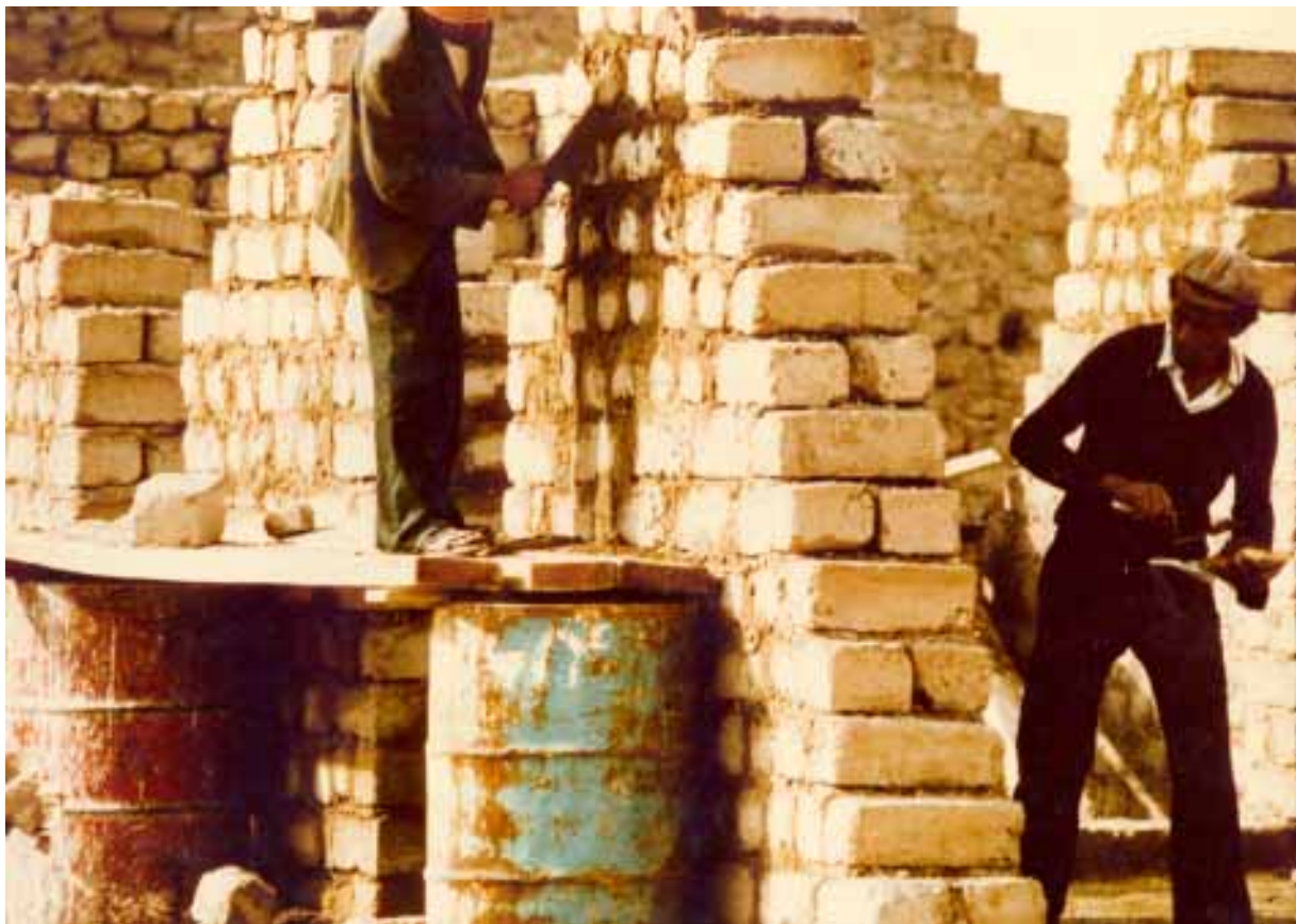
Stabilised mud bricks made by hand at first; later by machine press
