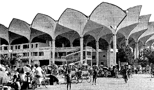
Kamalapur Railway Station, Dhaka.
