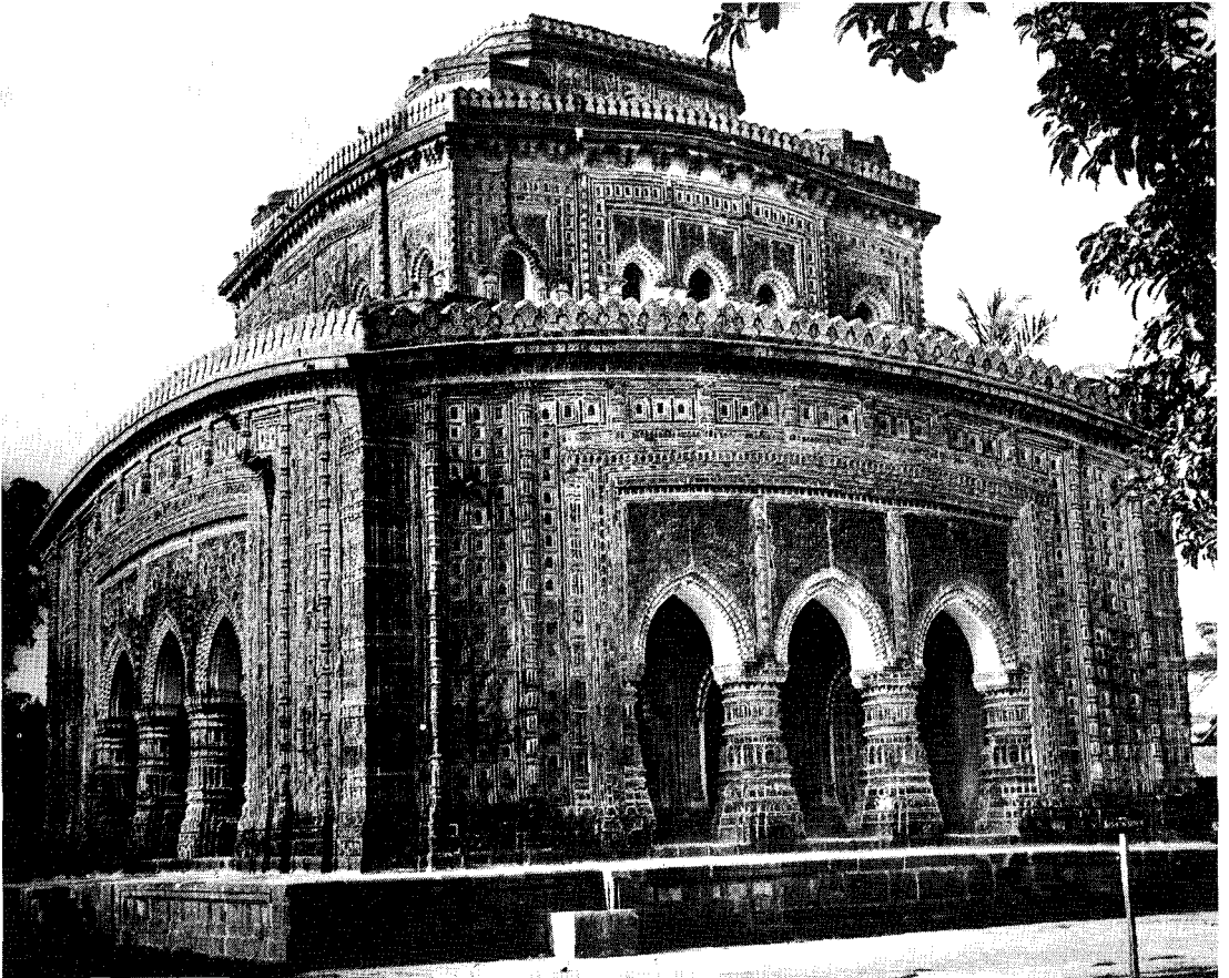
Kantanagar Temple, after repair of damage by earthquake in 1897 A D
