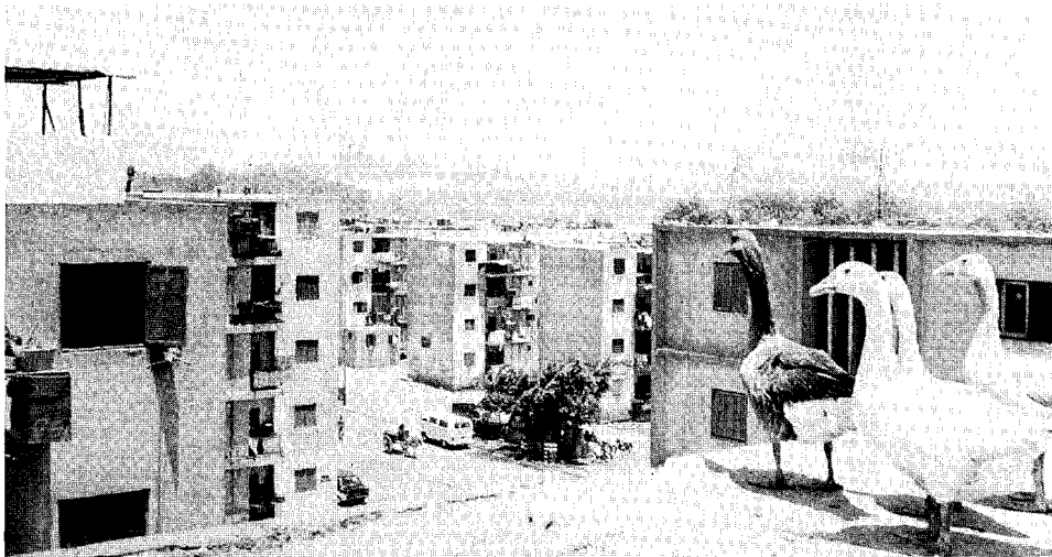
Inhabitants of the top floors of the mass housing project in Cairo keep animals on the rooftops. Access is via holes in the concrete roof.
