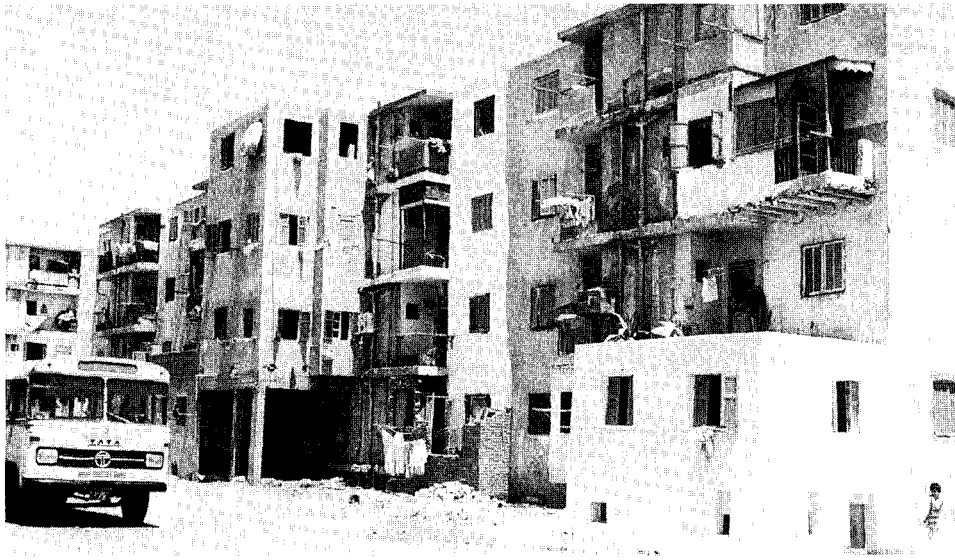
The same mass housing scheme in Cairo. The photograph shows the backs of the apartments, with extensions built illegally by residents. Note the four-story extension, indicating cooperation between occupants of different floors. This area was invaded by police charged with the demolition of illegal additions.
