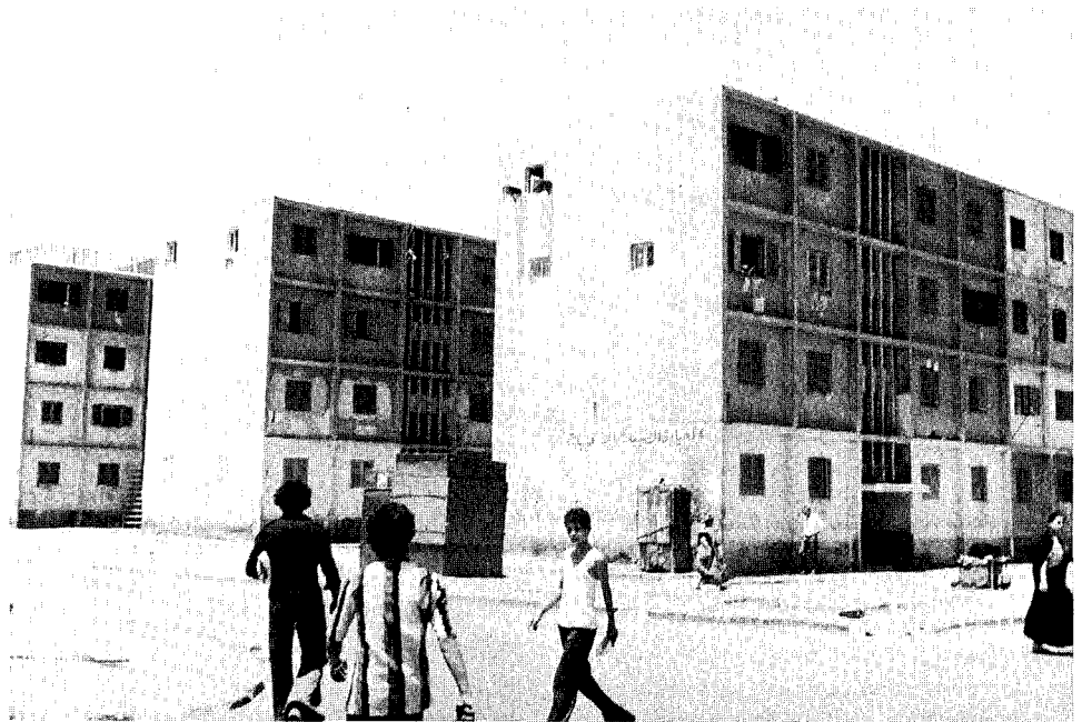
Mass housing project in Cairo, built of large concrete prefab panels
