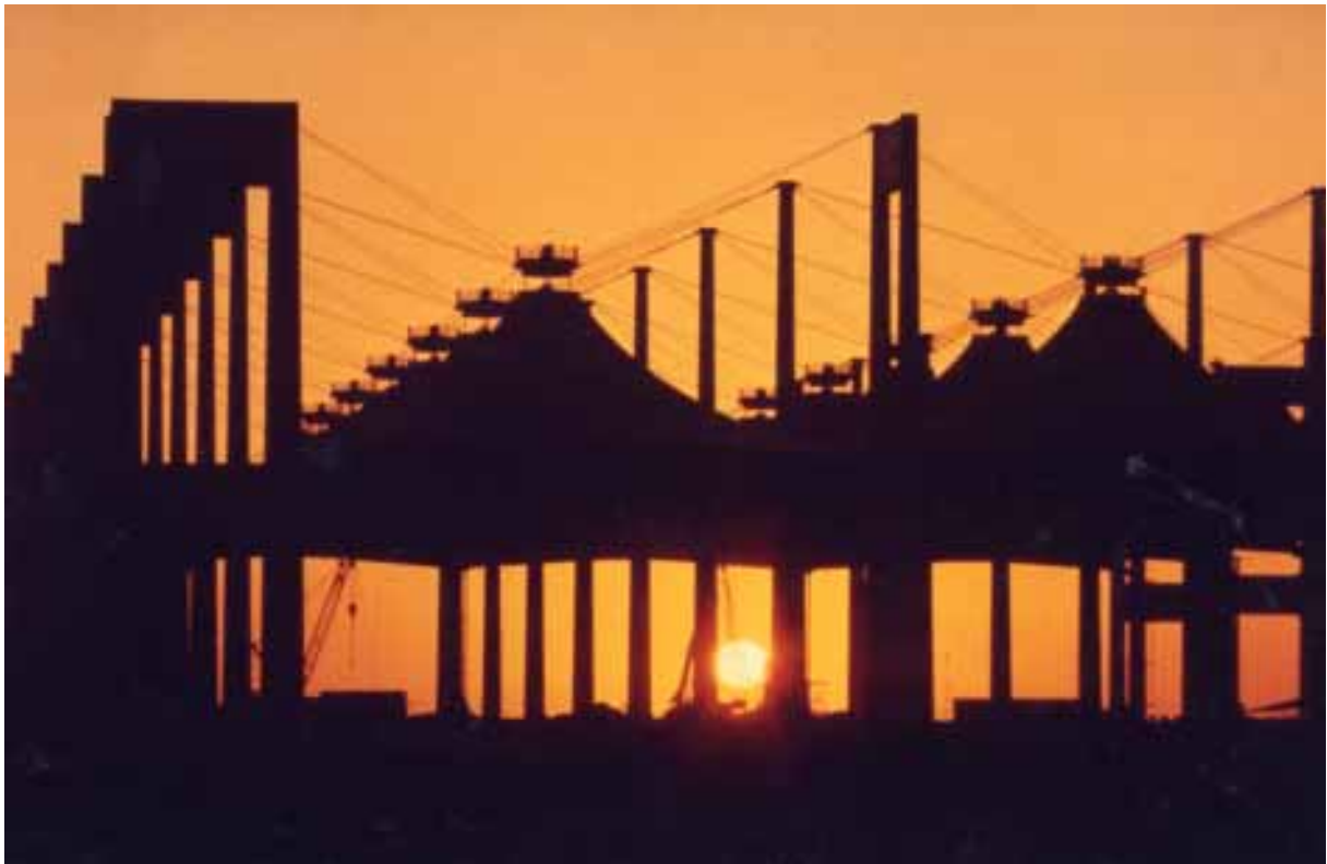
Using electronically synchronized equipment, the pre-assembled tent units were raised simultaneously
