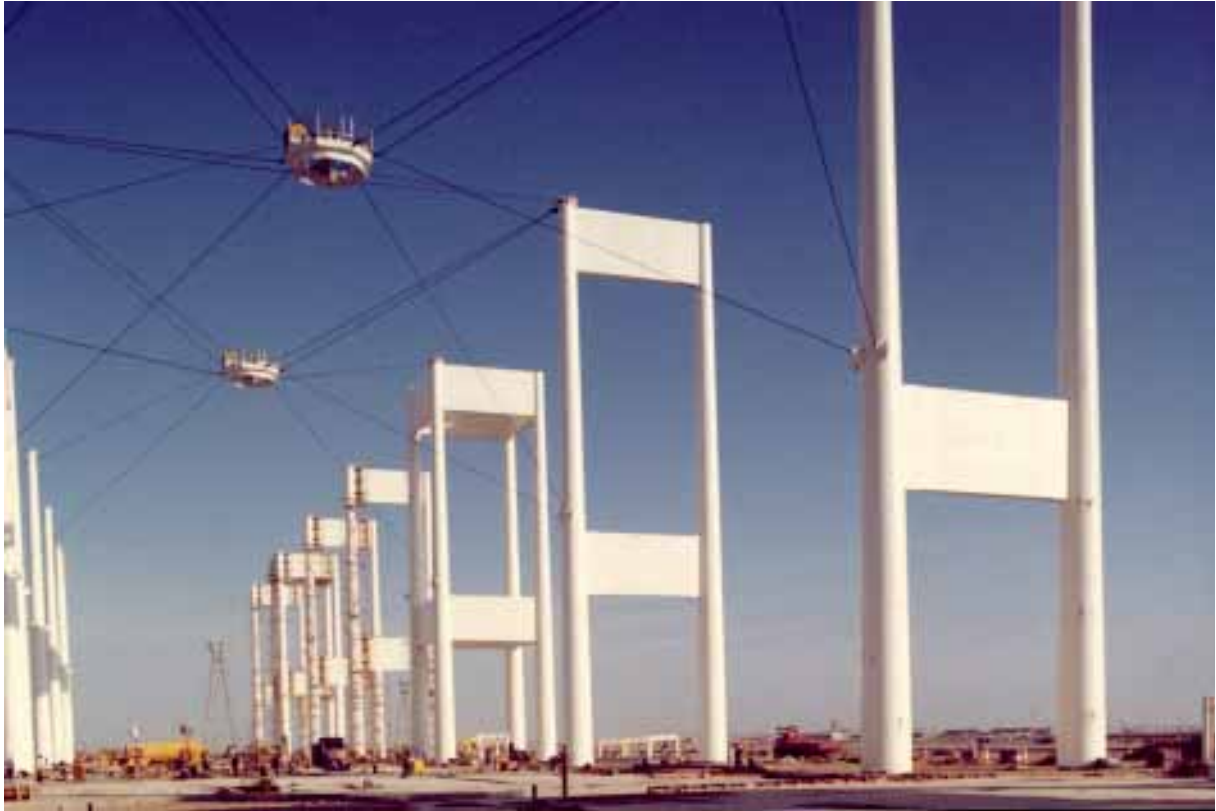
During construction: steel pylons and open tension rings
