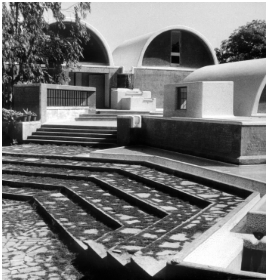
Main entry area; flat and vaulted mosaic tiled roofs; sunken areas with glass block ceiling lights
