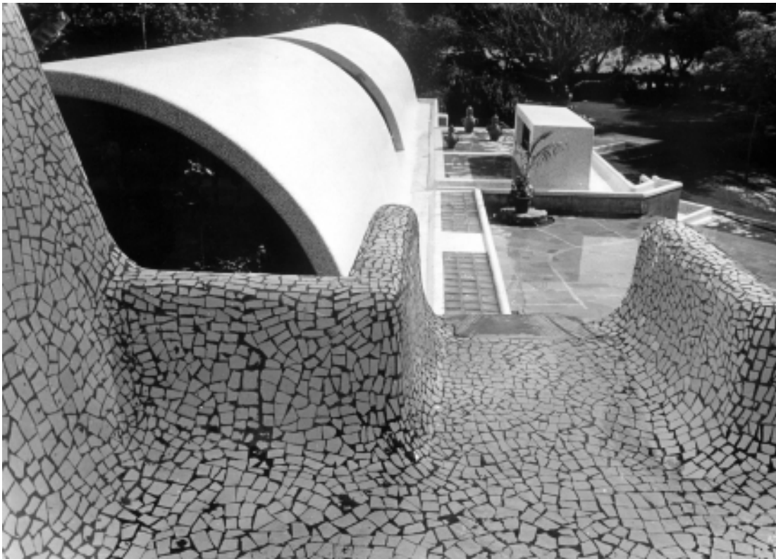
Recycled glazed mosaic tile chips; vaulted roofs divided for extra light
