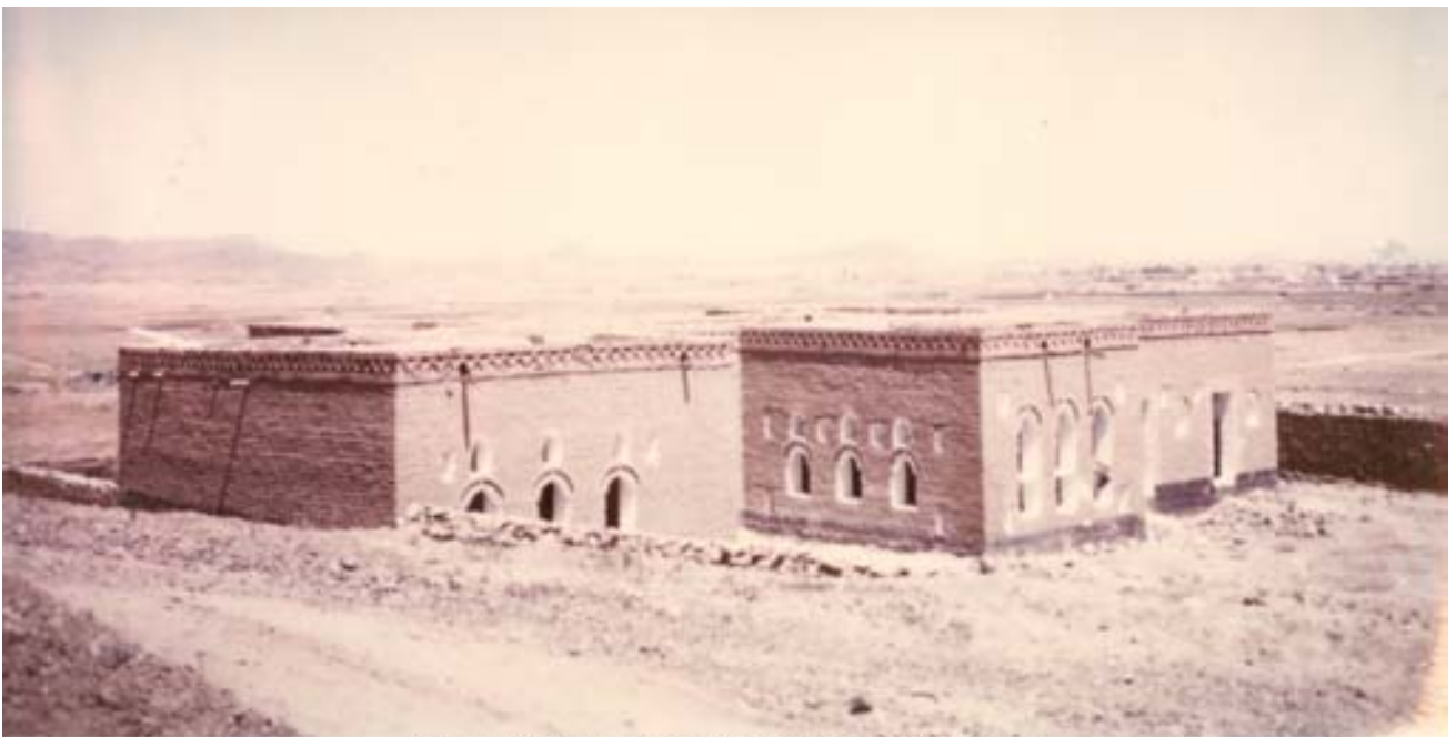
Construction photo: principal facade
