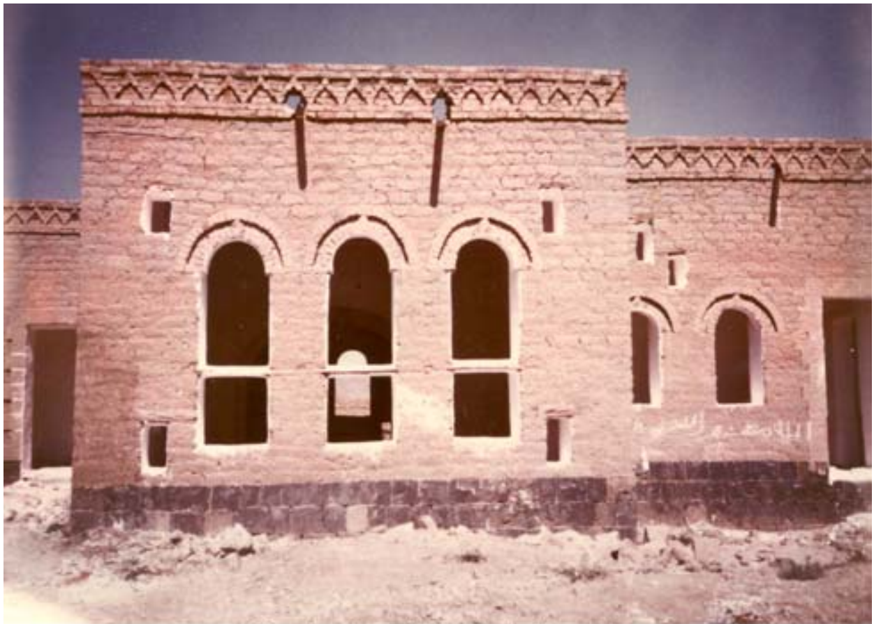
Construction photo: principal facade
