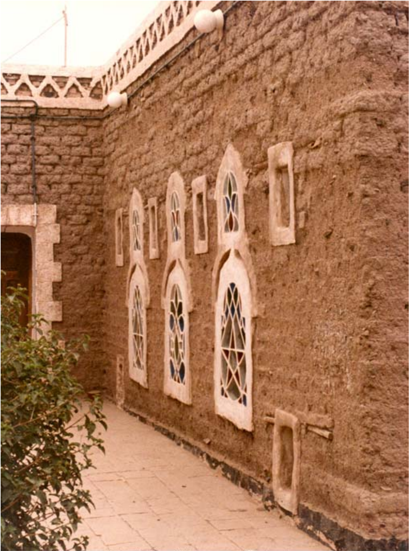
Entry (left) and living room side elevation
