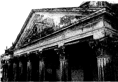
The north pediment, Ruplal's Block (western wing). The only such pediment in the structure, it highlights the most imposing of the three blocks built in the neo-classical style
