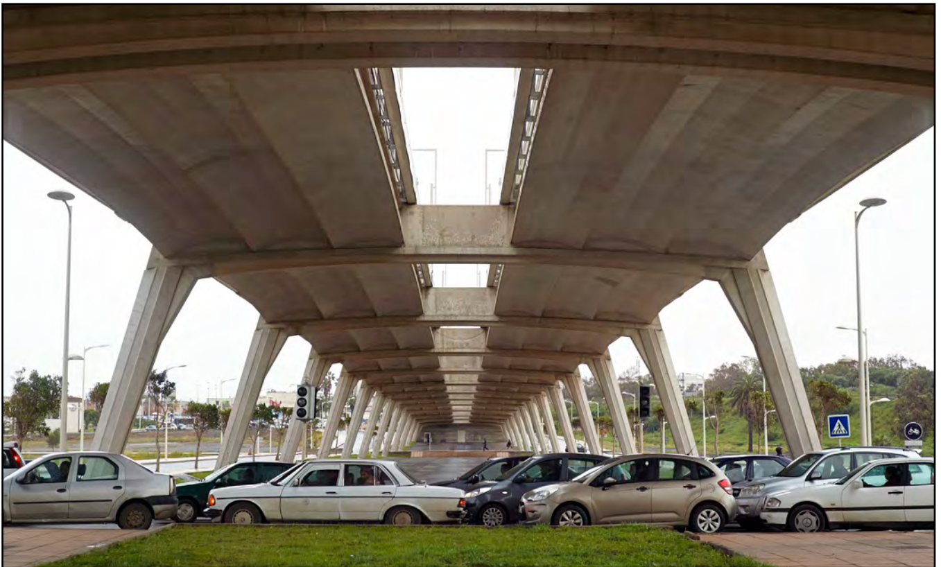
The Salé Viaduct is a simple repetitive structure with 28-metre spans of the same geometry.
