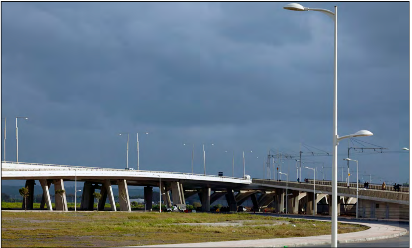
Nautical base bridge, on the Rabat bank, curves on plan while descending.
