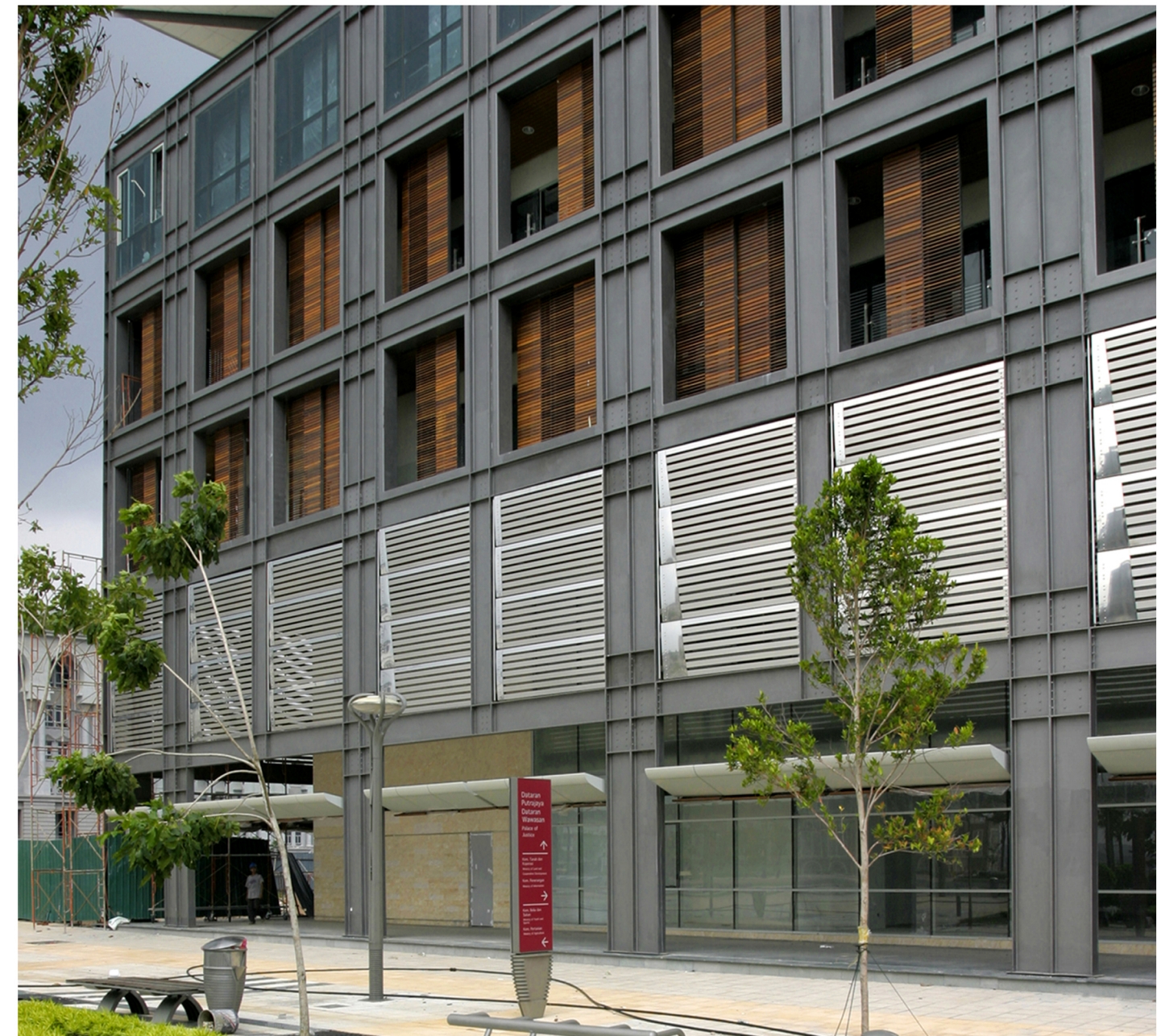
Front Facade - a screen of painted mild steel that creates a semi-transparent filter between the city and the building, a brise-soleil to diffuse glare and create shade.
