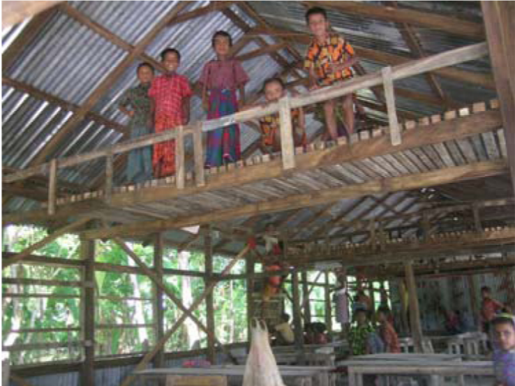
Construction of platform above 6.5 feet level and testing G.I. tension wires for structural load bearing capability.
