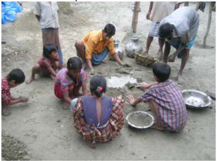
Active participation of family members during building cement-stabilized mud plinth
