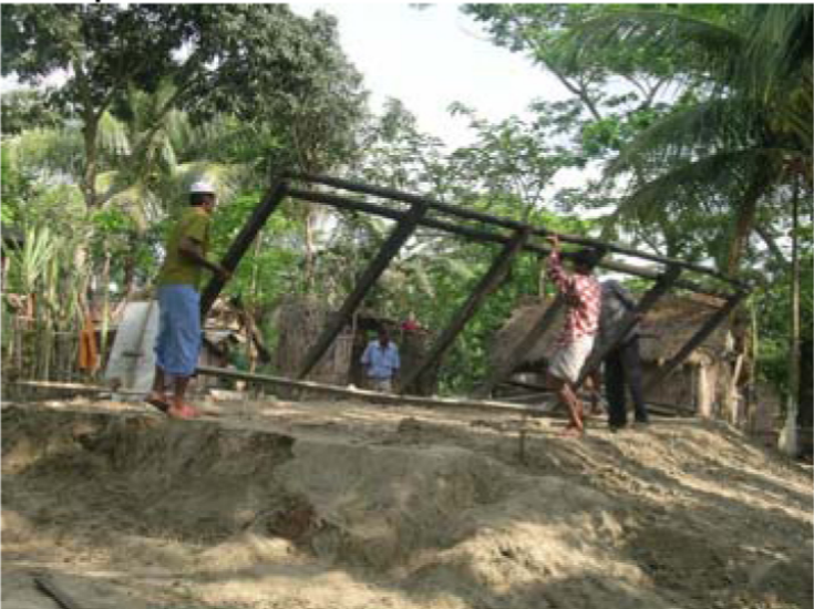
Dismantling existing house and recycling materials as much as possible
