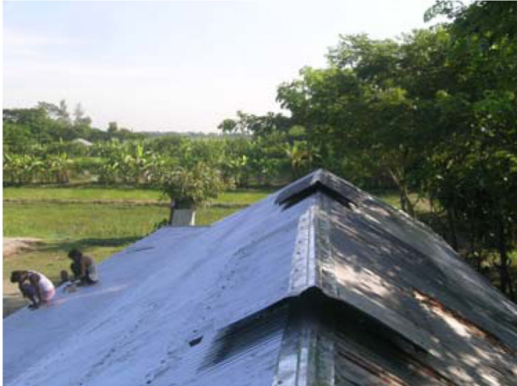
Ventilation roofs were constructed for venting the hot air outside
