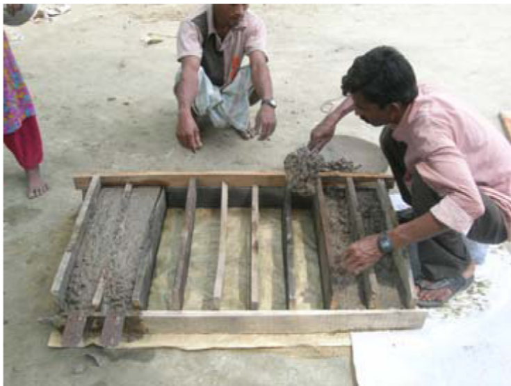
Making of concrete stump for damp-proofing base of wooden posts
