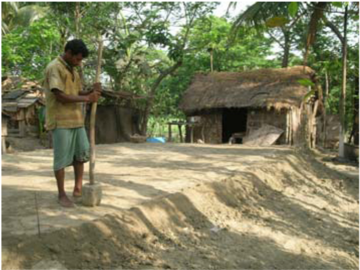
Ramming is important for earthen plinth
