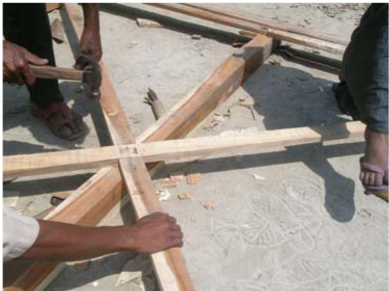
Horizontal and vertical cross-bracings make houses stronger
