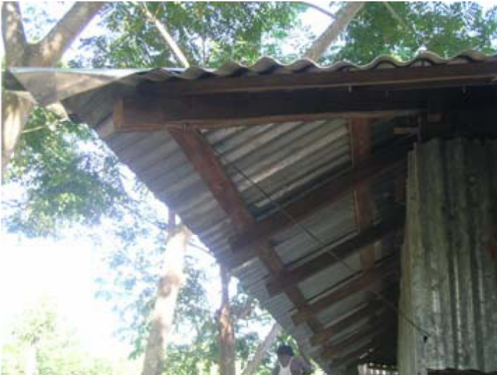
Tying the edge of roof with the posts to make it stronger against wind
