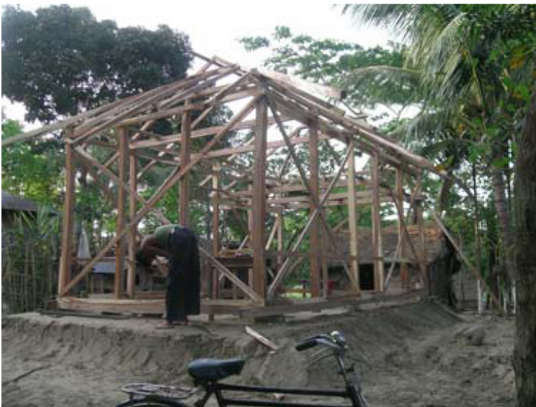
Erection of structure of house
