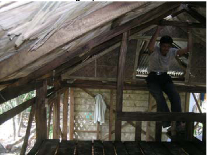
Construction of platform above 6.5 feet level (if possible, with recycled wood from the existing house)
