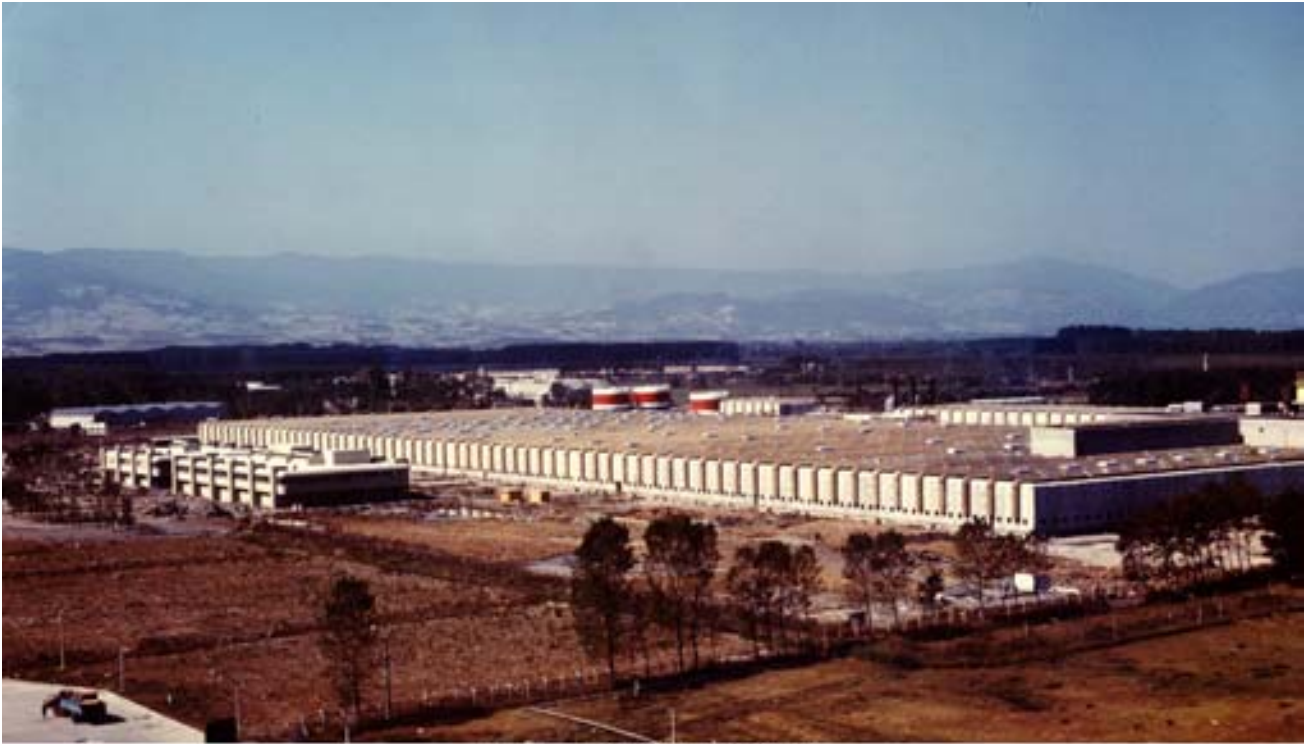
General view of plant
