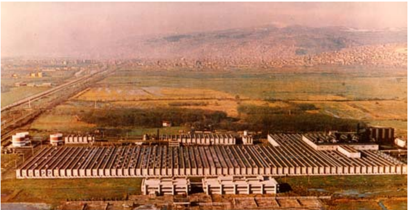
Aerial view of plant
