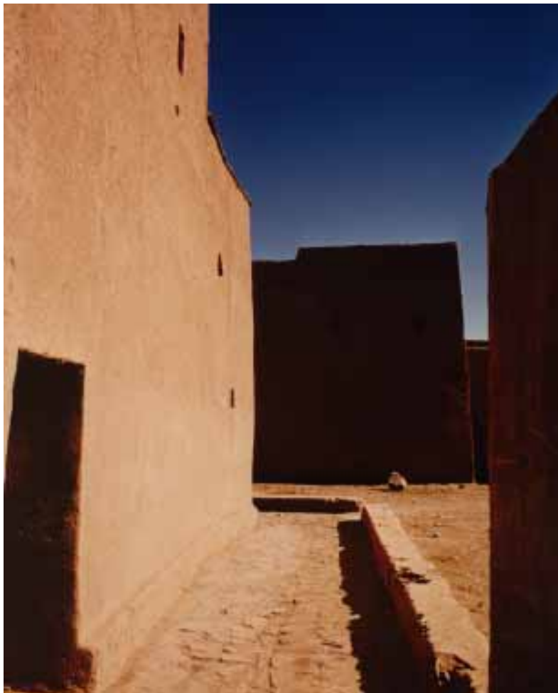
Demolition of houses in very poor condition, reconstruction, repair and resurfacing of the street in the Qsar of Tinezzouline
