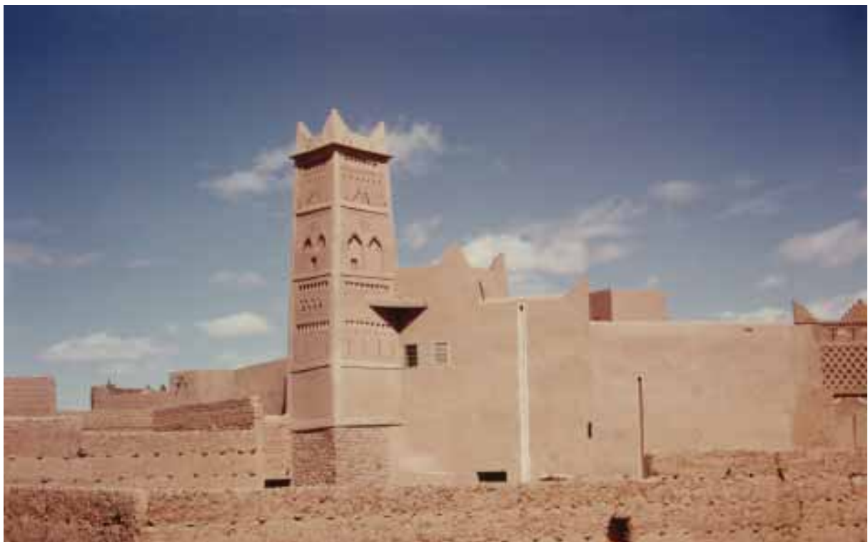
Restored 'borj' of a private house at Rbat Lahjar.
