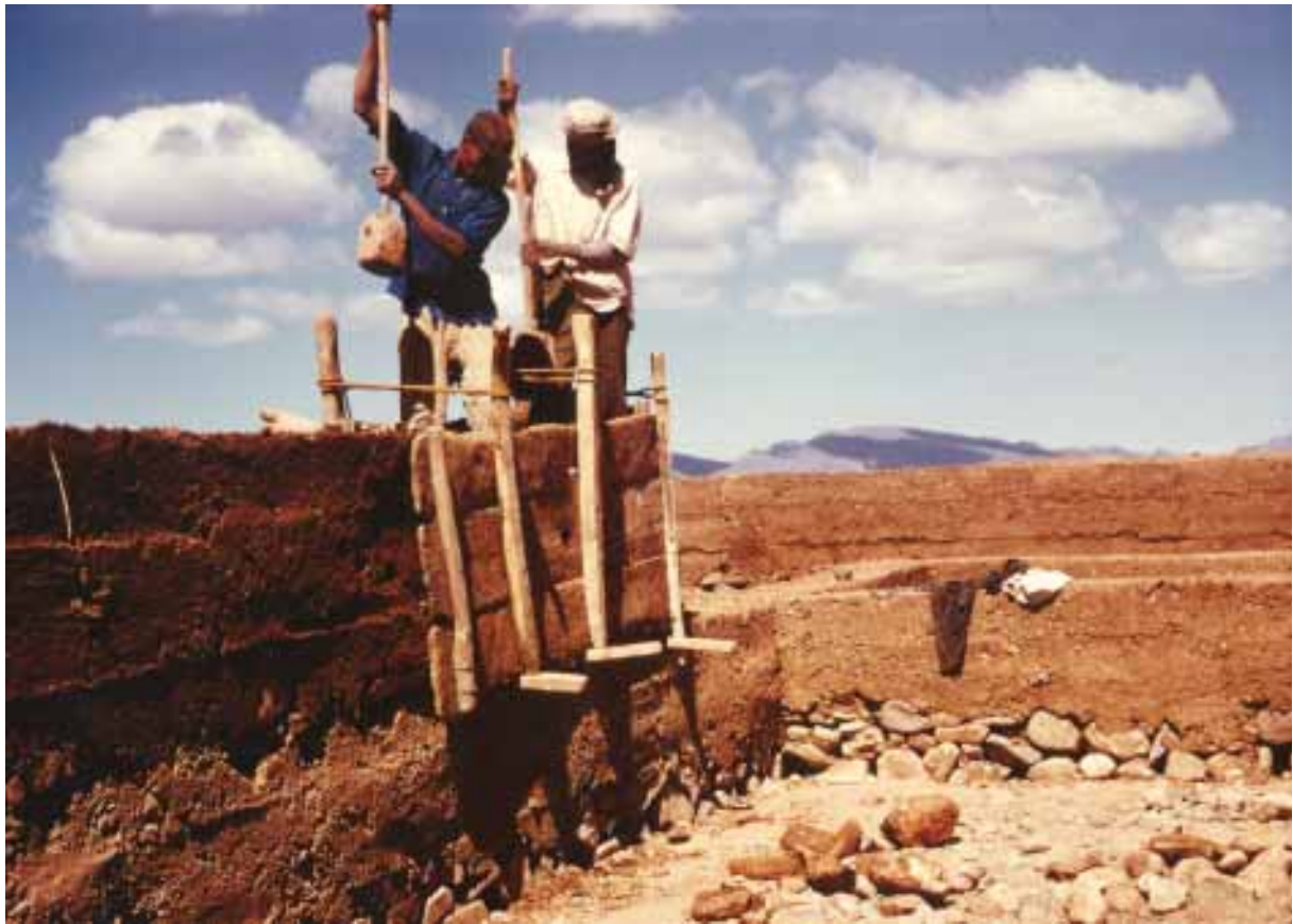
Execution of mud wall on stone base between two wal forms.
