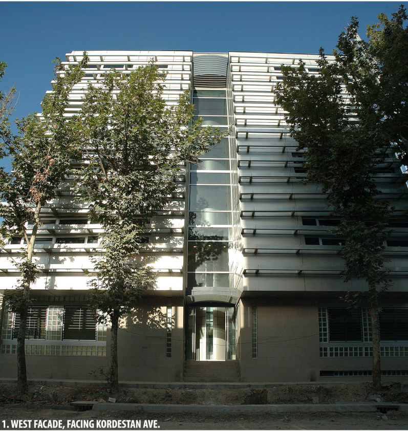
1. WEST FACADE, FACING KORDESTAN AVE.
