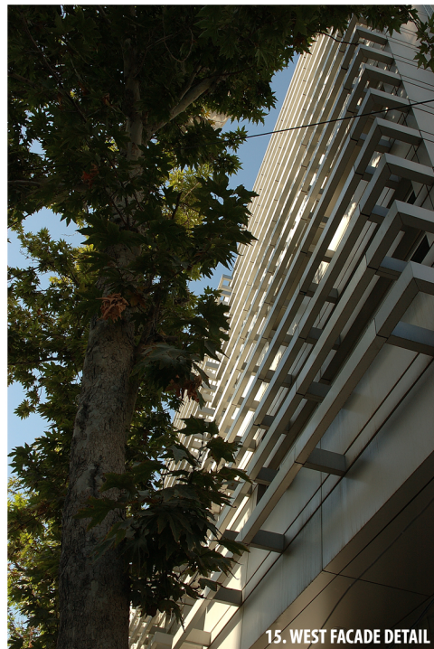
15. WEST FACADE DETAIL
