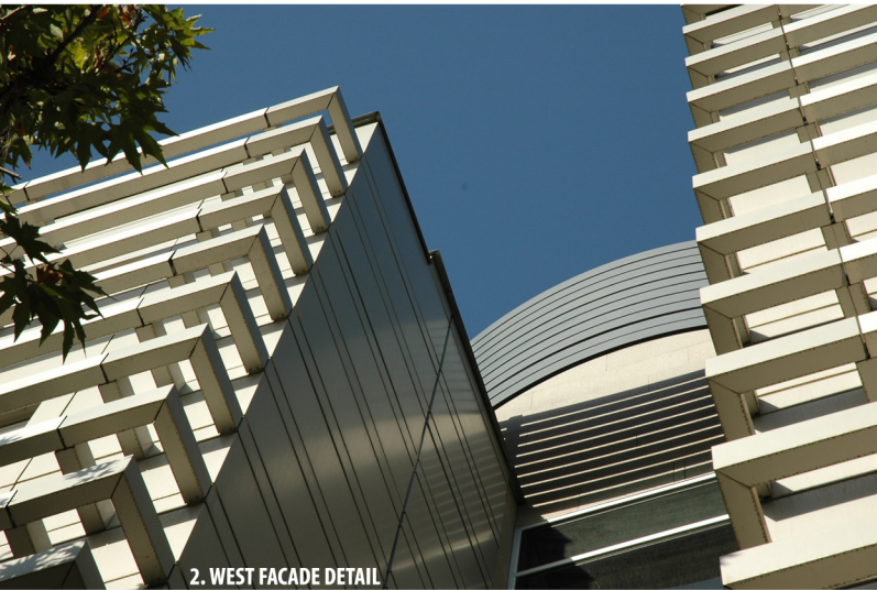
2. WEST FACADE DETAIL
