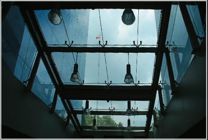
The ceiling of the Assembly hall
