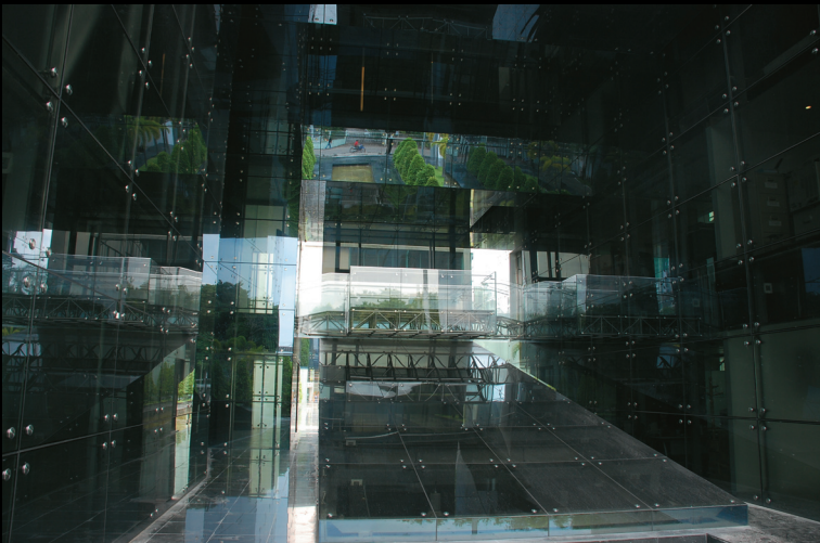
Building facade (view from the VIP entrance)
