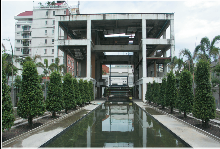
View from the under construction building
