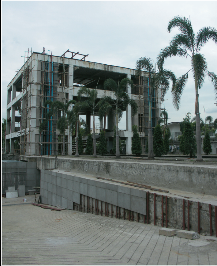
View from the under construction building
