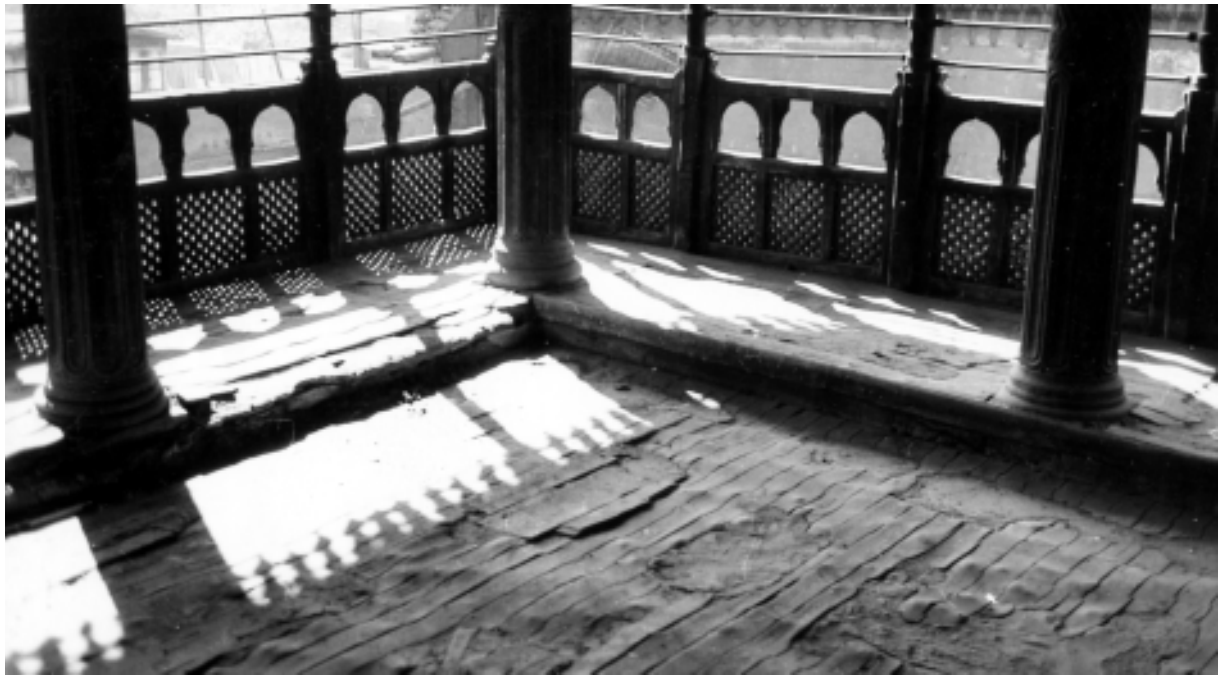
Sabil Kuttab: first floor before restoration
