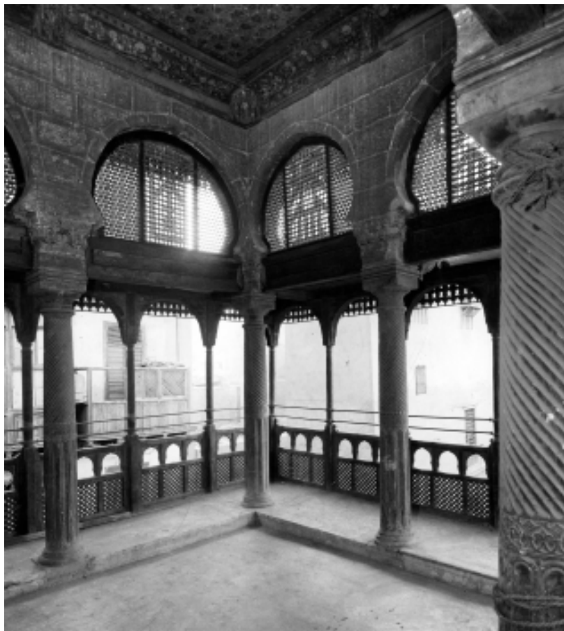
The first floor of Fountainhouse after rebuilding and consolidation
