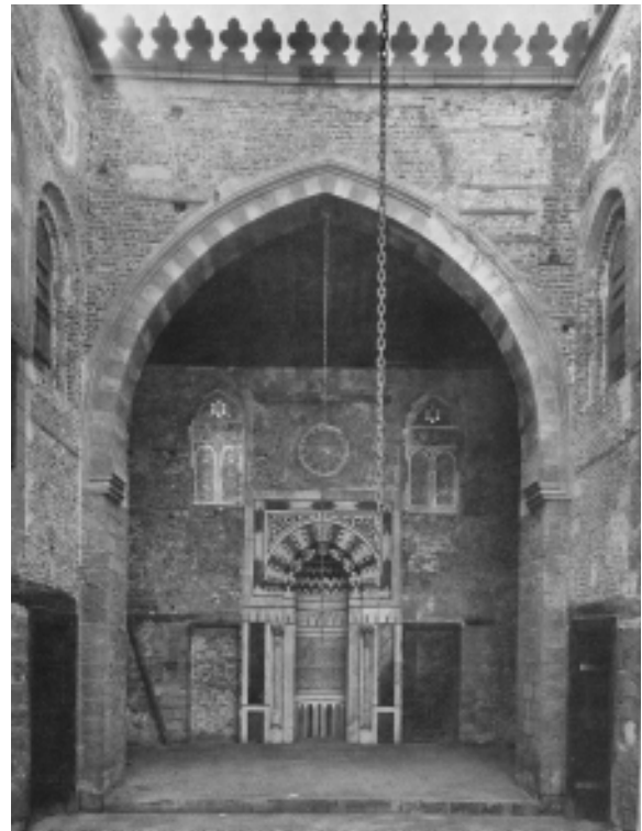
The main "iwan" after restoration. Note the reintroduction of parapets.
