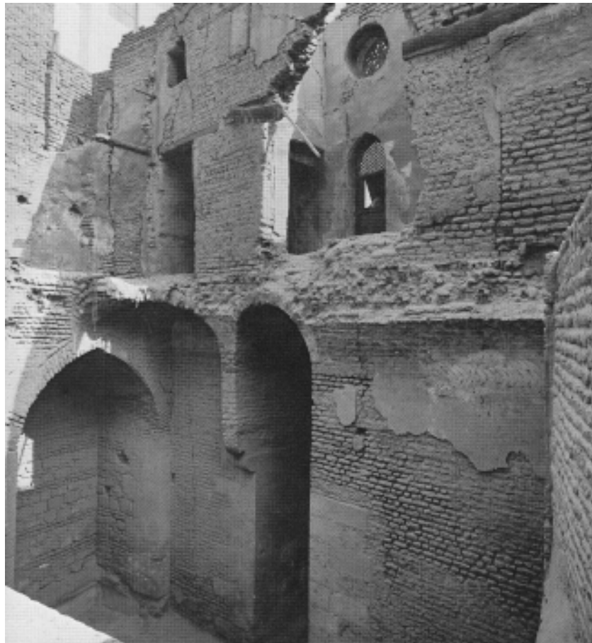
South wing of Madrasa before restoration
