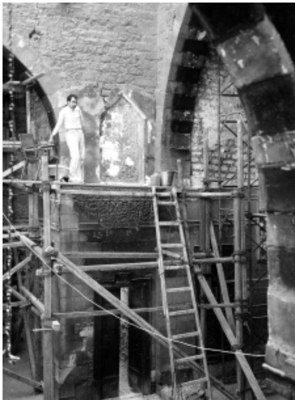
Madrasa Tatar al-Higaziya: repair and stucco
