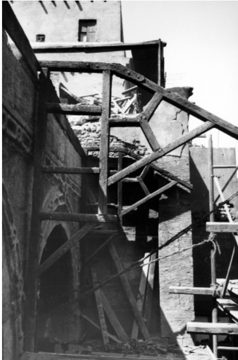
Sabil Kuttab: repair of roofing
