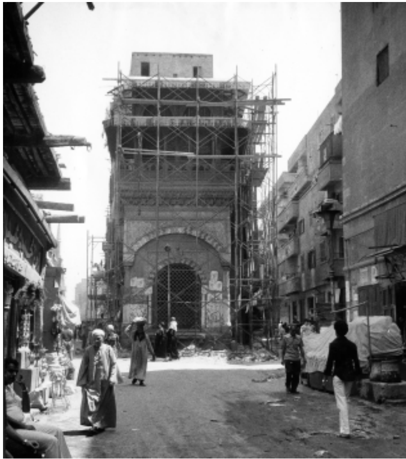
View on Fountainhouse during restoration of the roof
