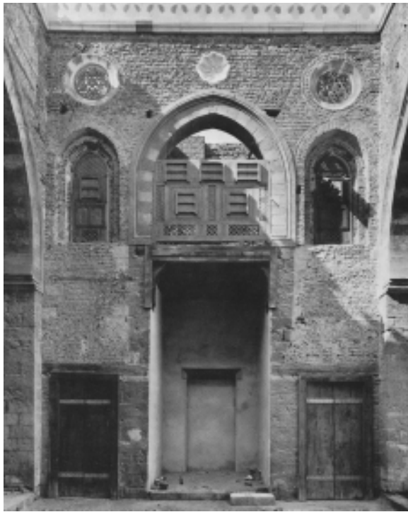
The north “iwan” with the old Mahrabiya before restoration
