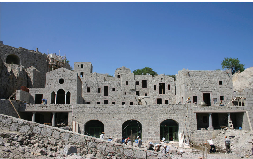
Construction of the Row Houses
