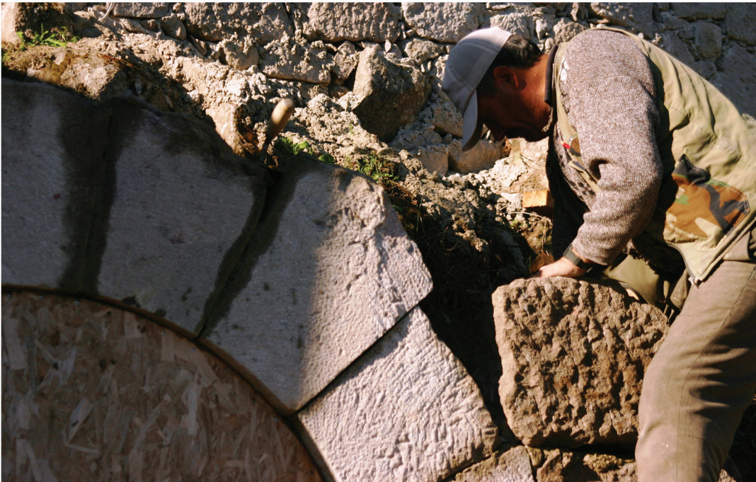
Construction of a Stone Arch
