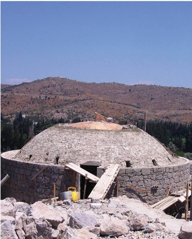
Construction of the Cistern
