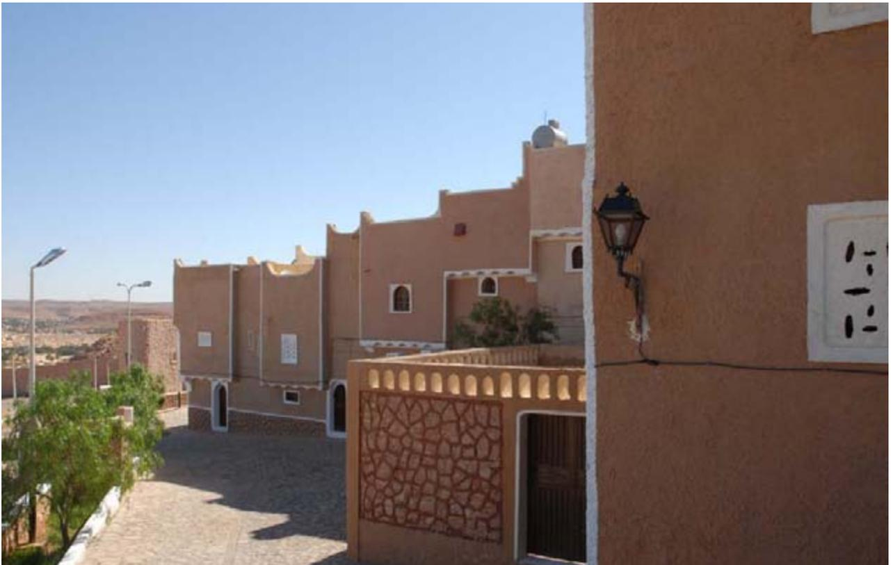
Exteriors of the buildings are made of lime, sand and concrete, only needing care every five years at little cost.
