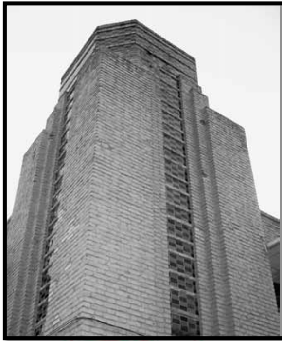
Figure 1. The Exterior detail (stair-case shaft) from a house in Abadan. Image scanned from the book: “Domesticity and Consumer Culture in Iran: Interior Revolutions of the Modern Era.”
