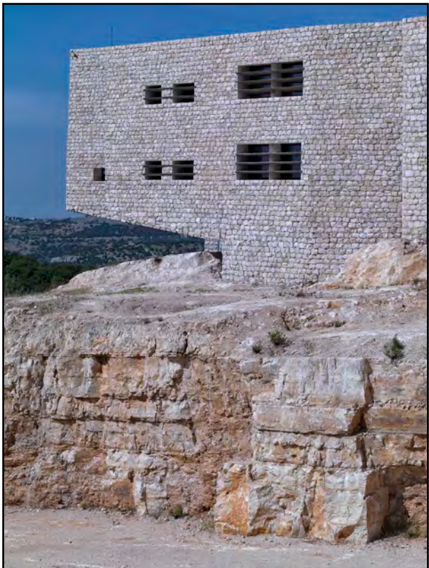
The southern facade absorbing most of the sunlight is fairly uniform in its stone skin broken by a few deeply cut windows and vertical incisions. In some windows, exposed tapered concrete louvers mitigate solar gain
