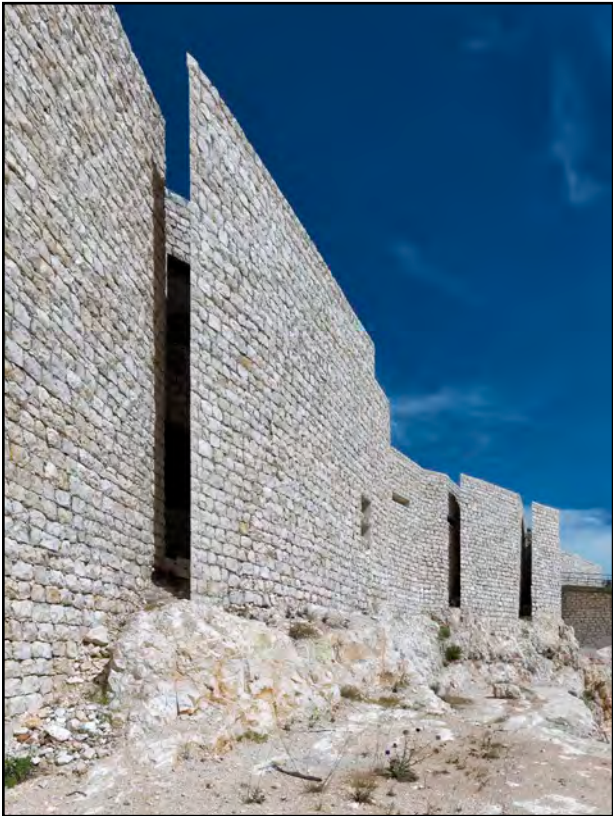
The southern facade absorbing most of the sunlight is fairly uniform in its stone skin broken by a few deeply cut windows and vertical incisions. In some windows, exposed tapered concrete louvers mitigate solar gain
