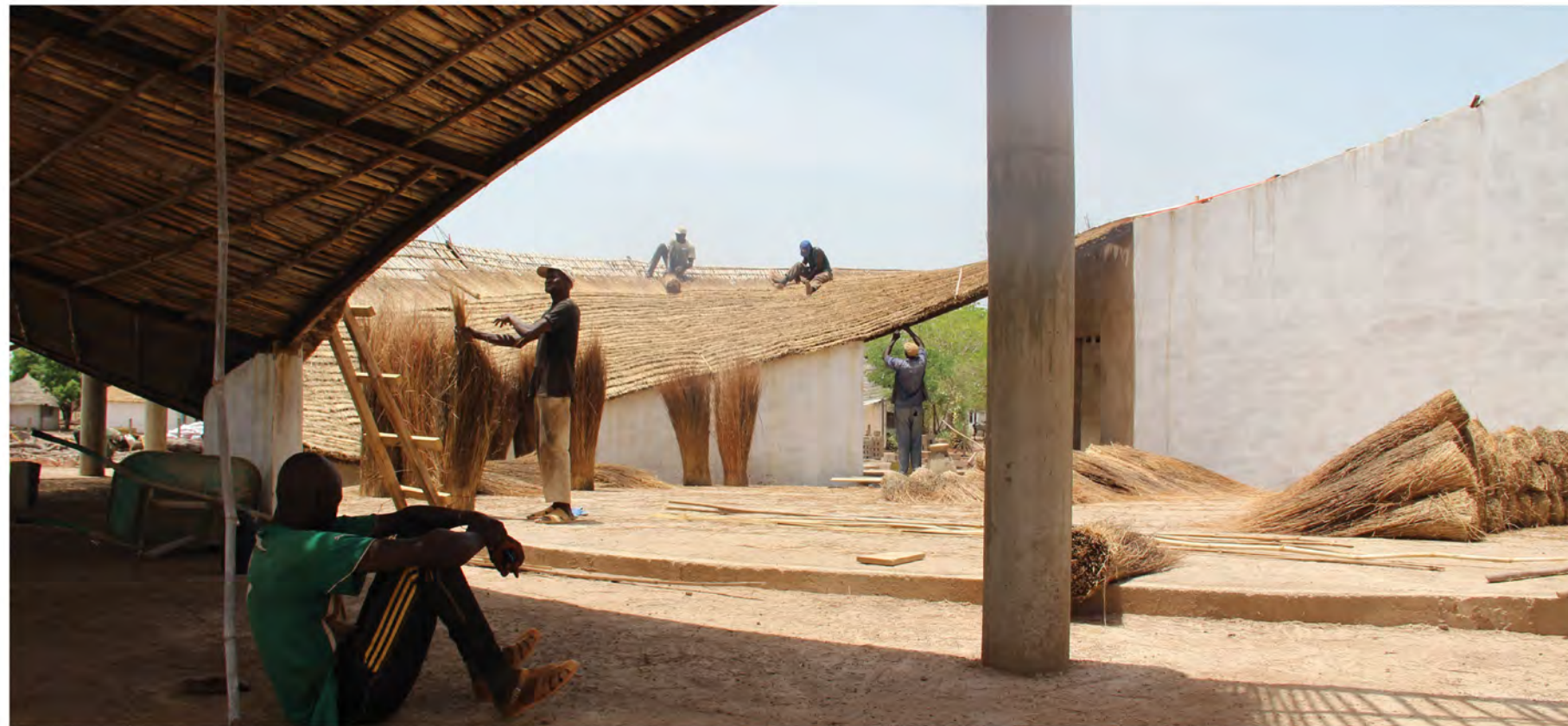
Images (Clockwise from top right): Local villager with thatch used for the roof; Magueye Ba, village doctor, overseeing construction of Thread; children on site during construction; construction team applies layers of thatch to the roof.
