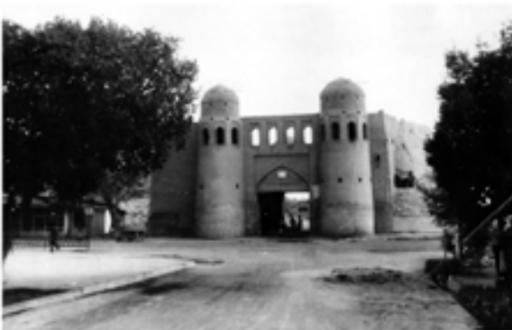
b) Bagha Dervasa, after restoration.
