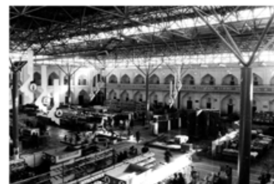
43) Caravanserai, used as trade centre - roof structure.
