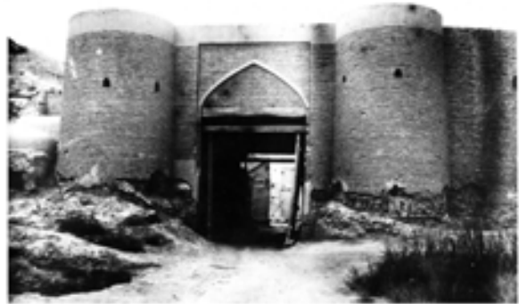
c) Tash Dervasa, during restoration.
