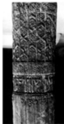
c) Djuma Mosque, during restoration.
