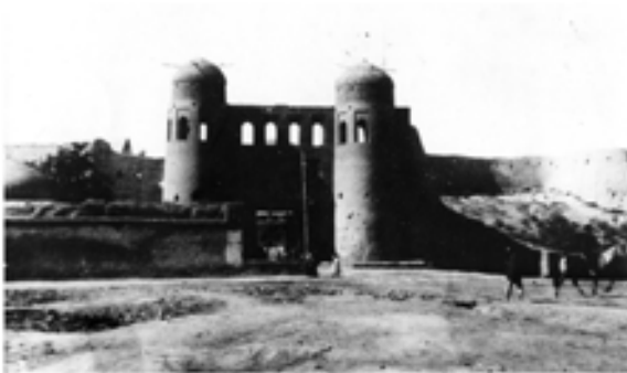
a) Bagha Dervasa, before restoration.
