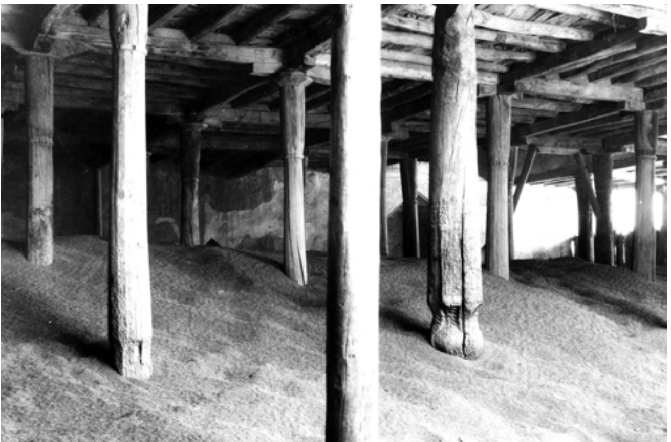
Djuma Mosque,before restoration
