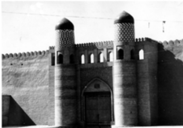
b) Kaspia Ark gate, after restoration.
