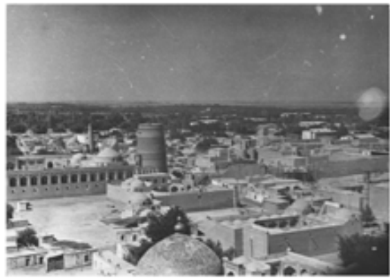
c) Fortress wall, before restoration.
