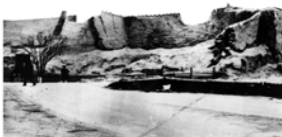
a) Aia Darvaza, before restoration.
