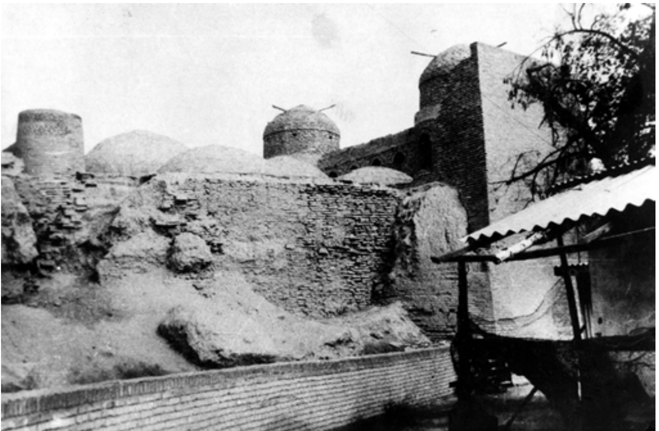
Bagcha Darvaza, during restoration
