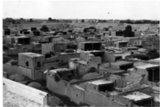
d) Fortress wall, nearby houses.
