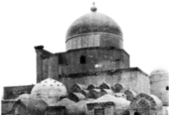
c) Pahlavan Mahmud Mausoleum, after restoration.
