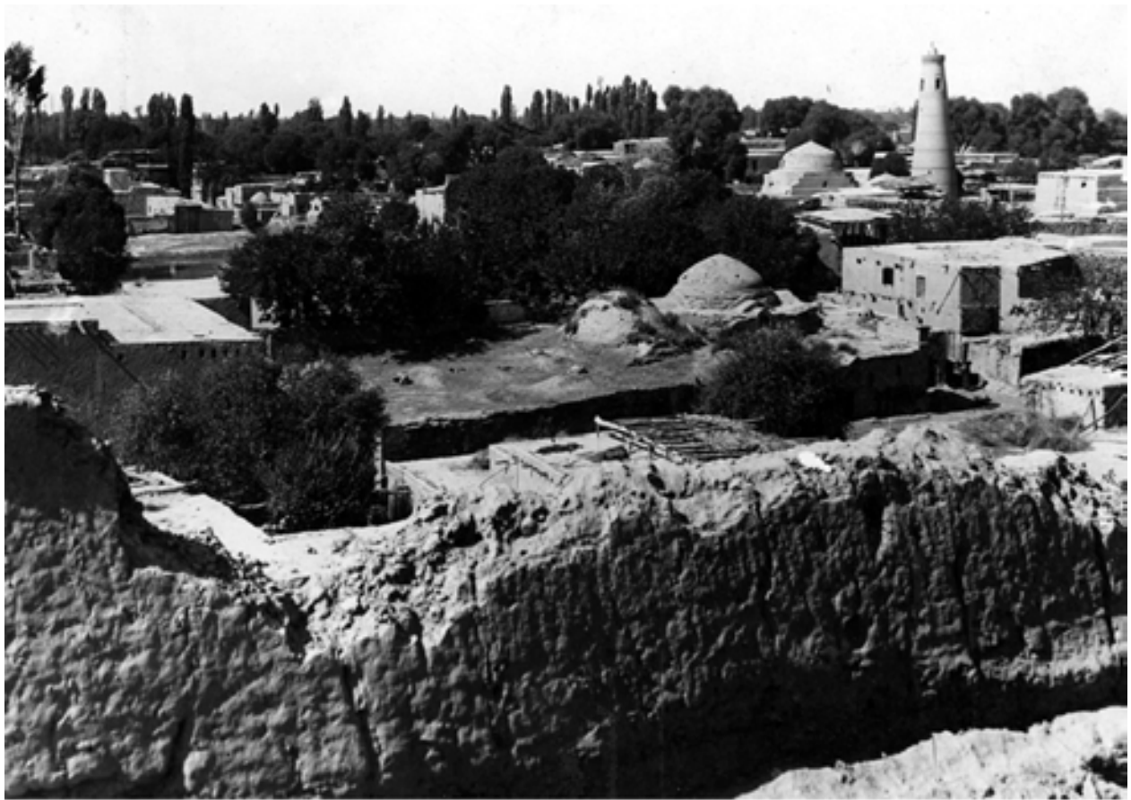
Fortress wall, before restoration
