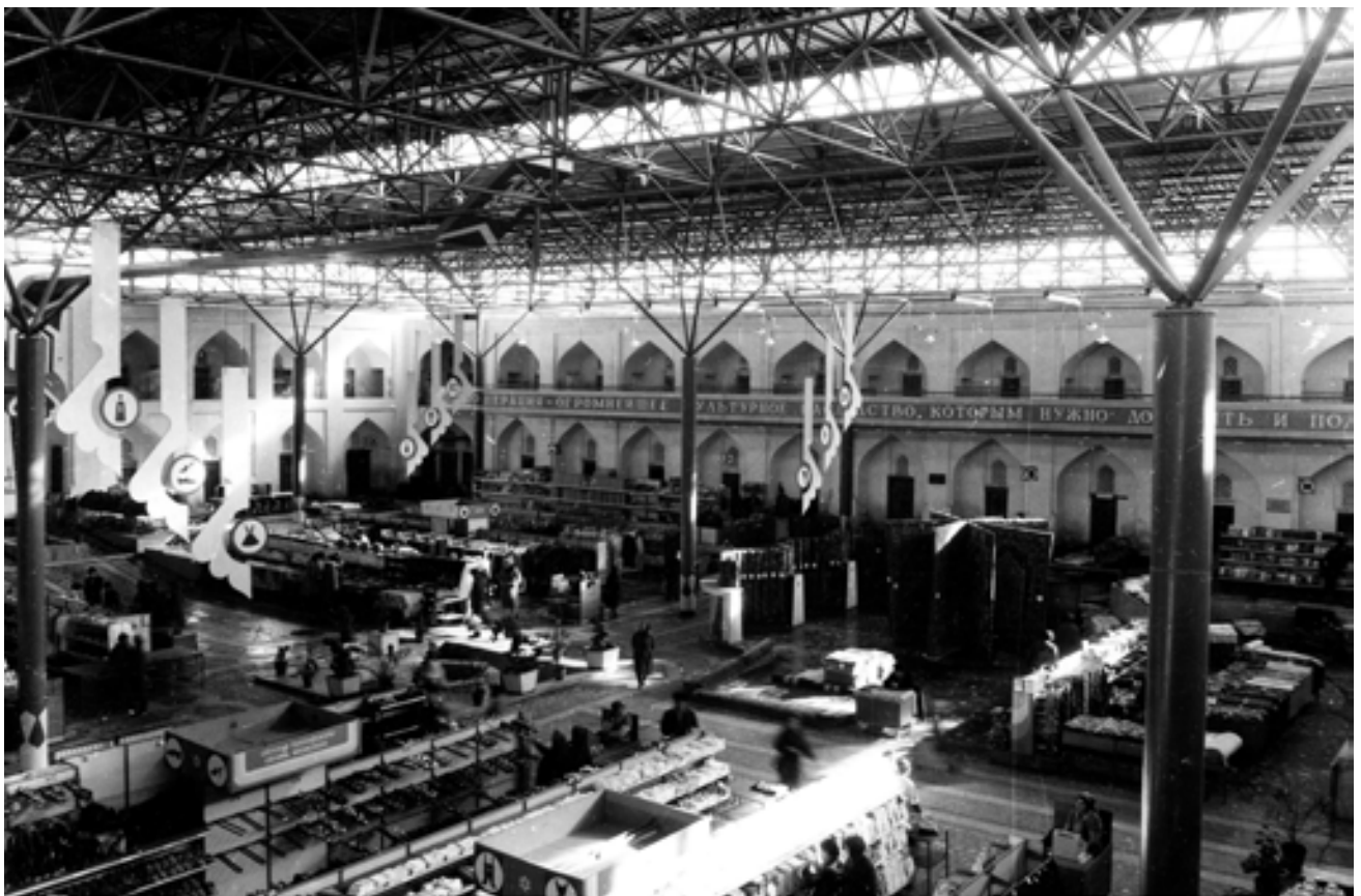
Caravanserai, used as trade centre - roof structure
