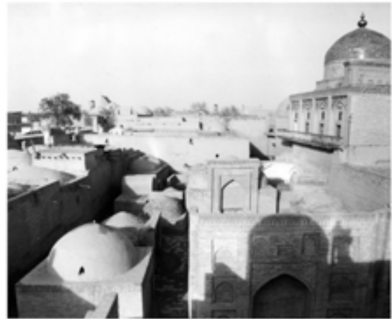
c) Complex near Pahlavan Mahmud Mausoleum, after restoration.
