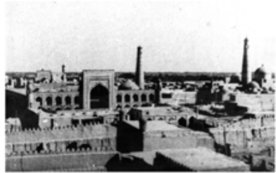
c) Kaspia Ark gate, general view.
