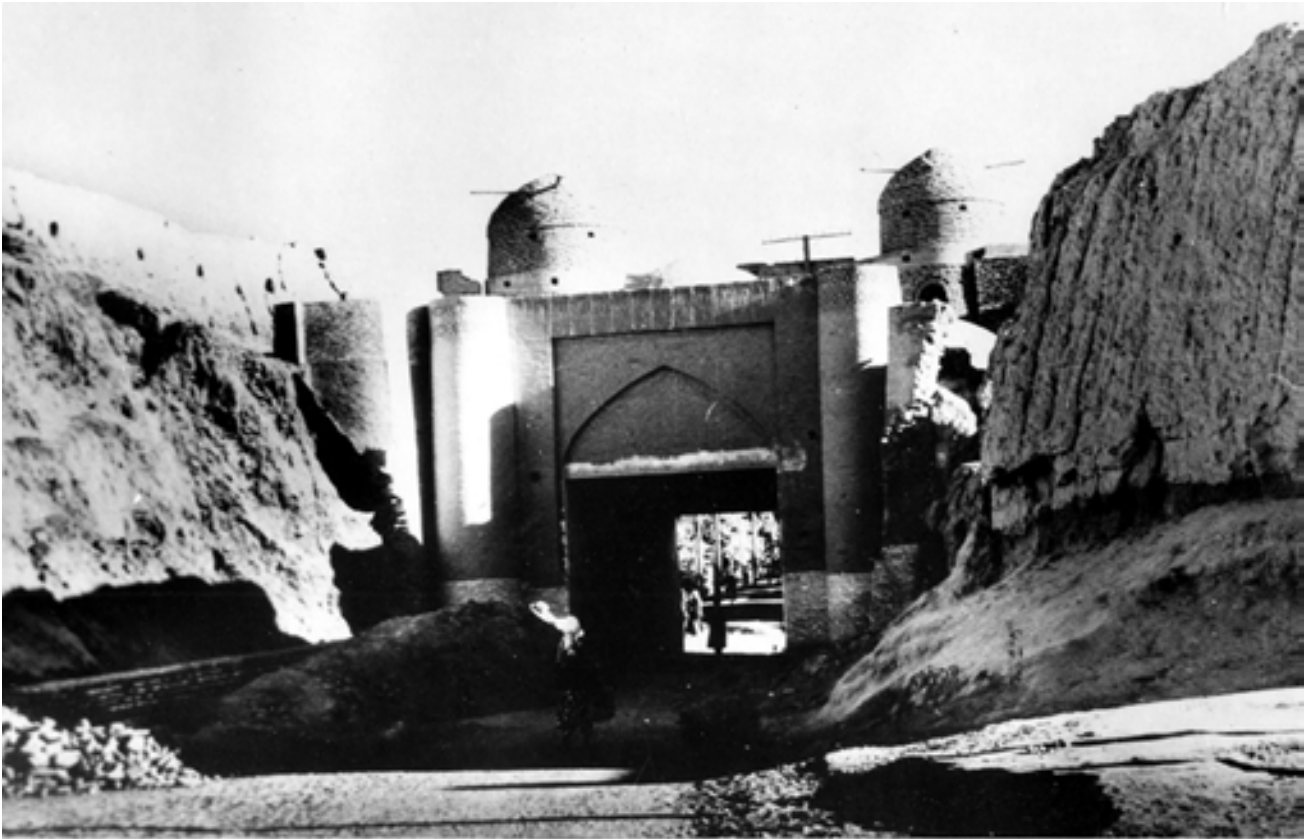
Bagcha Darvaza,during restoration
