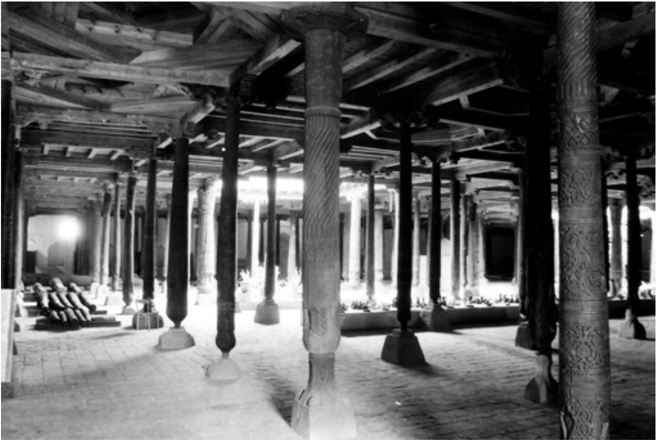
Djuma Mosque,during restoration
