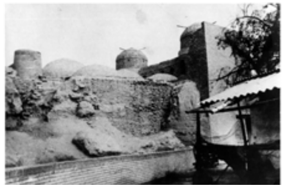
c) Bagha Dervasa, during restoration.
