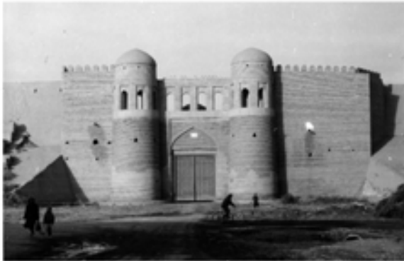
b) Tash Dervasa, after restoration.
