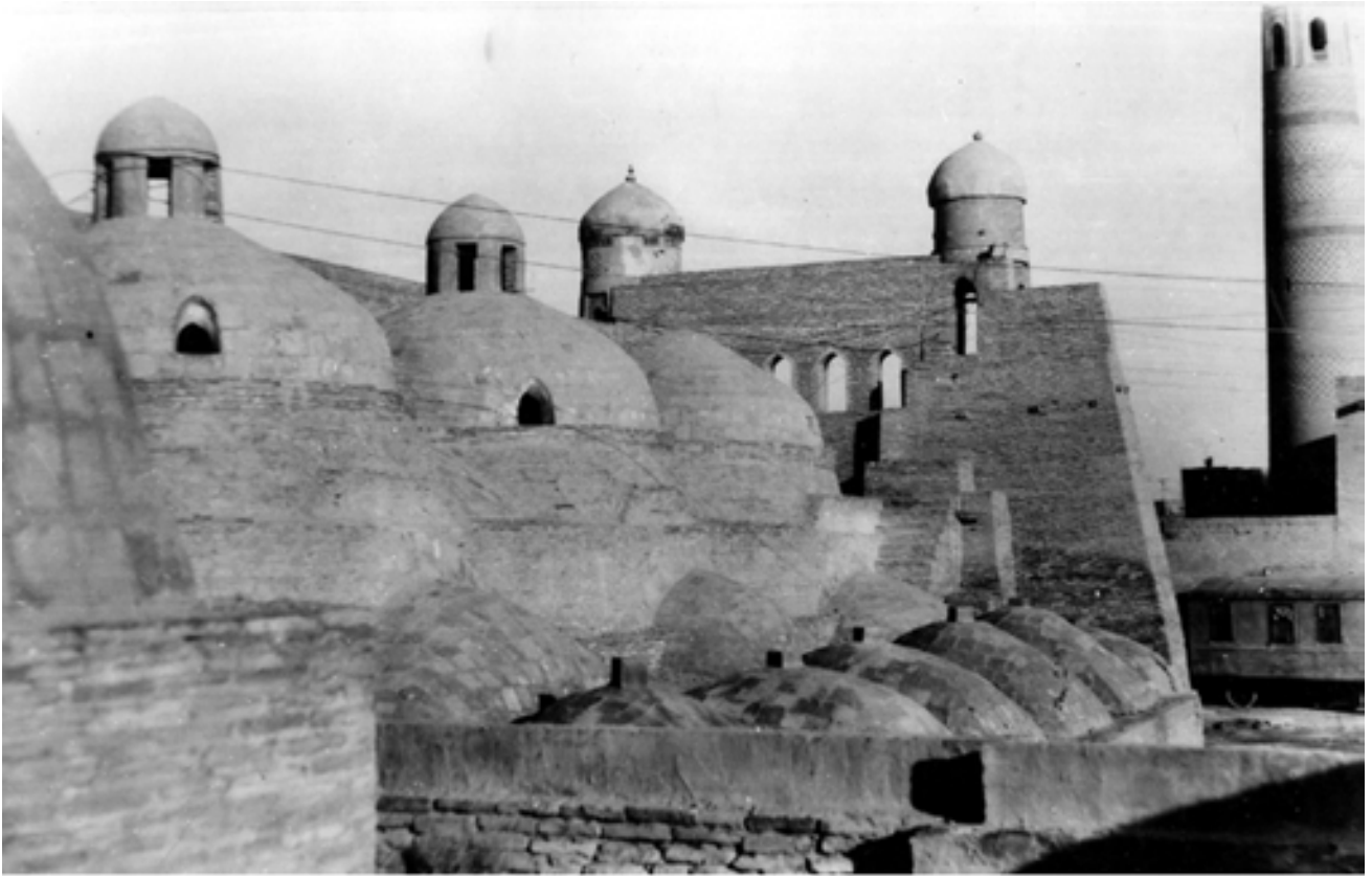
Palvan Darvaza, after restoration
