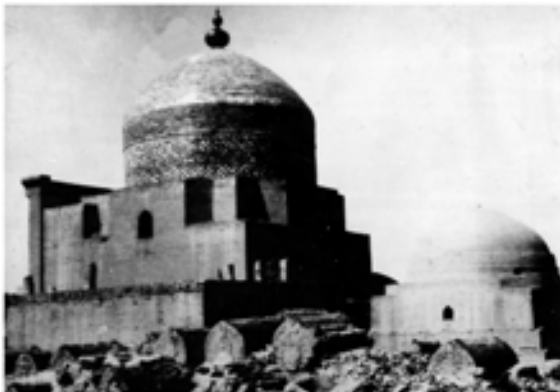
a) Pahlavan Mahmud Mausoleum, before restoration.
