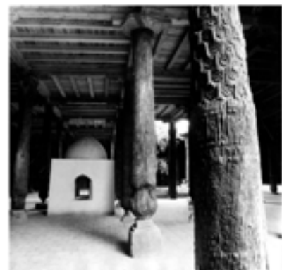
e) Djuma Mosque, after restoration.
