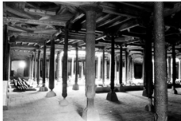
d) Djuma Mosque, during restoration.
