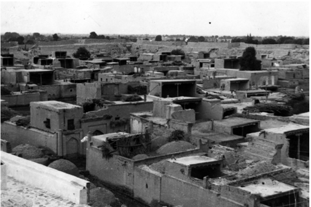
Fortress wall, nearby houses
