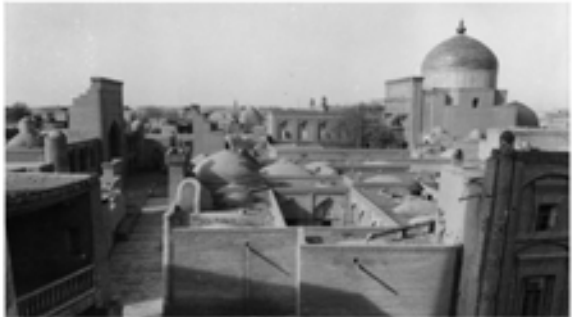
d) Complex near Pahlavan Mahmud Mausoleum, after restoration.
