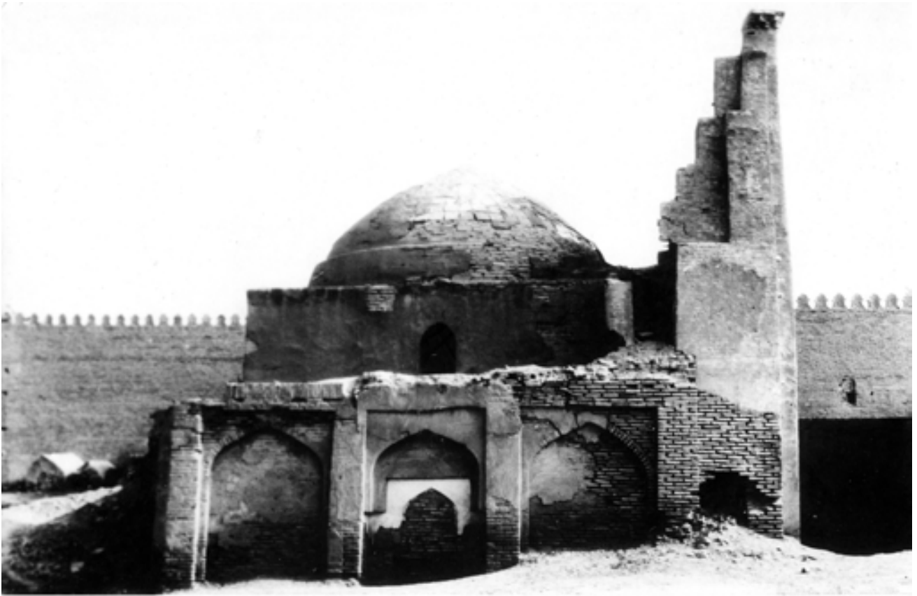
Uch Avliya Mausoleum, before restoration
