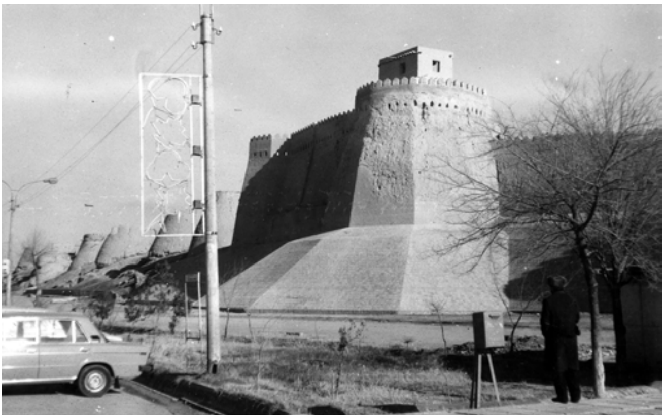
Fortress wall, after restoration
