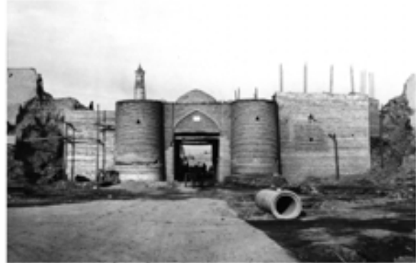
d) Tash Dervasa, during restoration.
