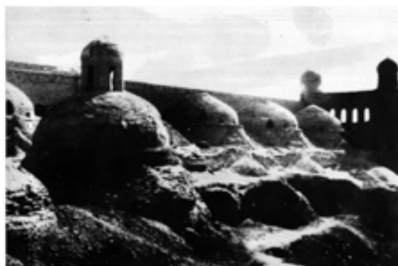
c) Palvan Darvaza, before restoration.
