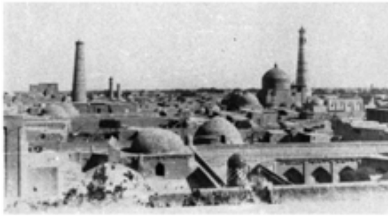
a) Complex near Pahlavan Mahmud Mausoleum, before restoration.
