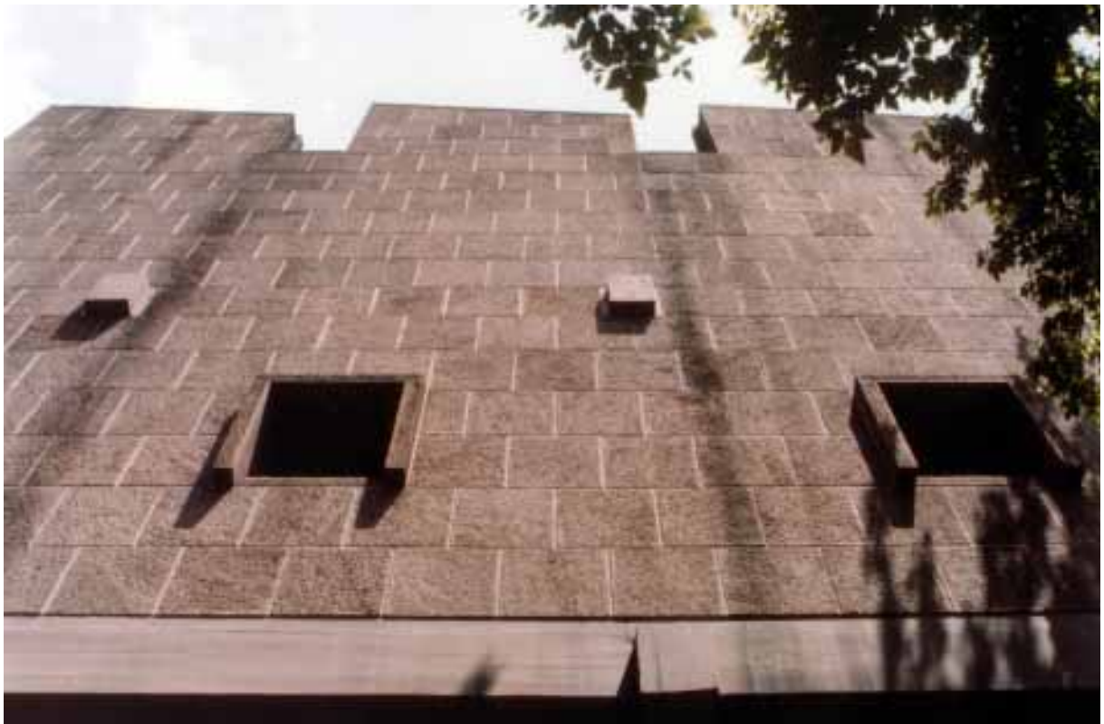
Partial view of library elevation. Red Ankara stone infill
