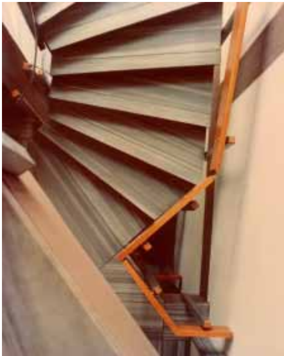
Detail of stair construction and finish
