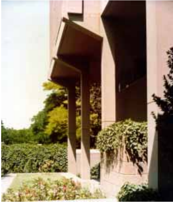
Structural skeleton of reinforced concrete
