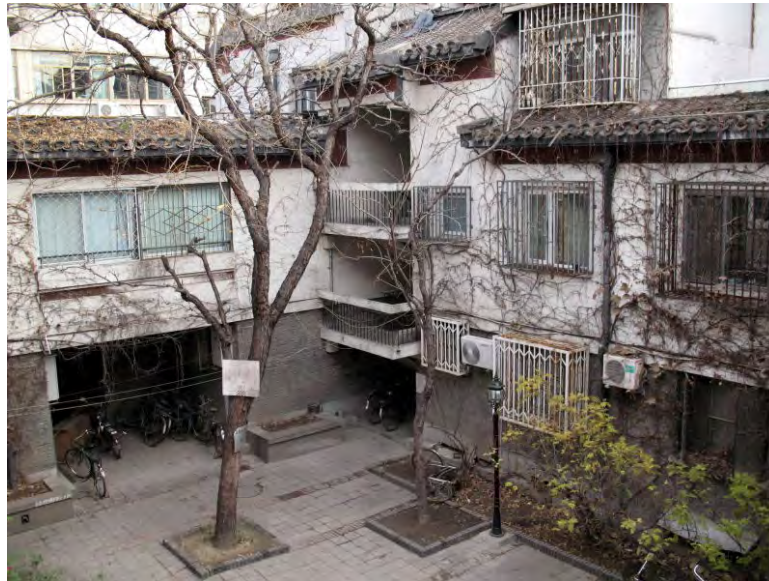
Figure 10. A new courtyard at Juer Hutong (Source: Author).
