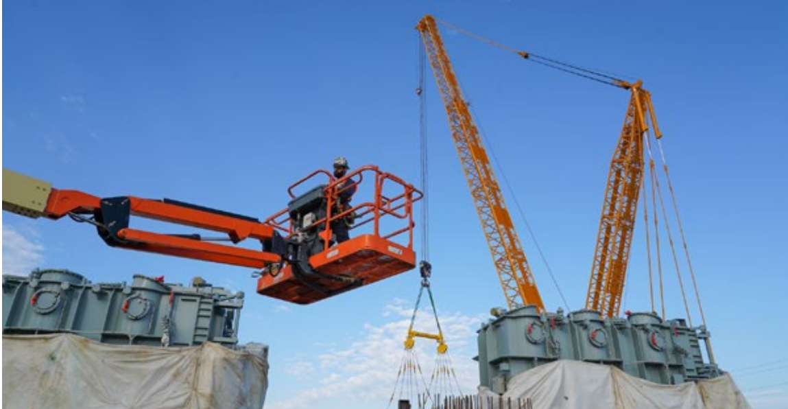
Construction at the Heartland Petrochemical Complex in September 2019.
