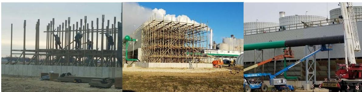
The new beer-degasser should be complete in the next couple of weeks. It is installed between the beerwell and the beer column to reduce the entrained CO2 in the beer. This will improve vacuum levels while we reduce summer time vacuum capacity constraints. It also reduce beer column carryover and allows for additional beer column throughput. This helps to reduces the cleaning frequency for the side stripper and will lower acidity in the alcohol.
